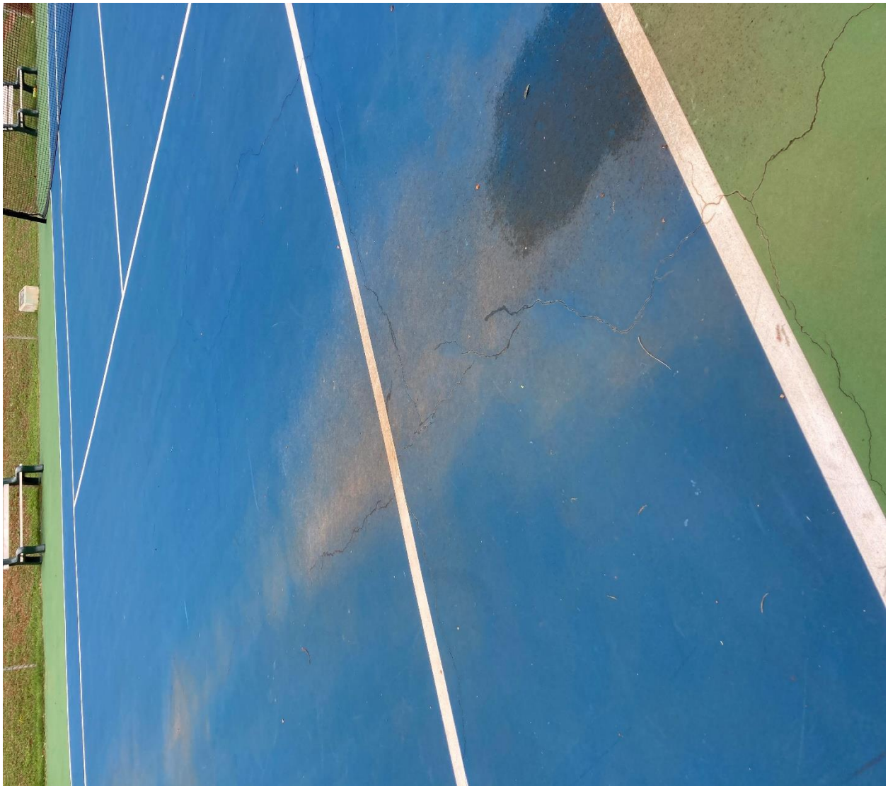
Tennis Courts Cracks in Surface Before
