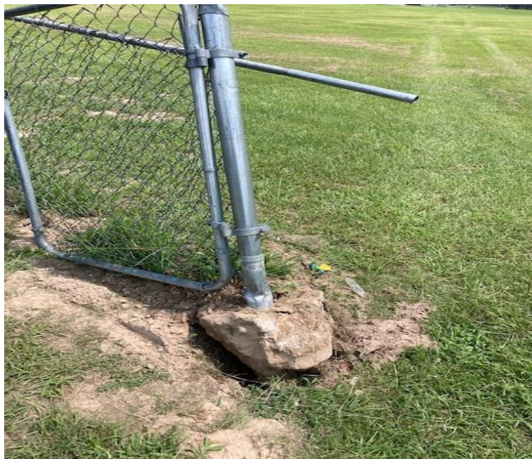
Damage to gate Pole Complex
