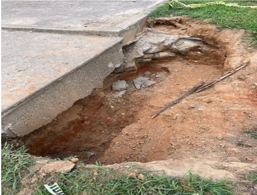
Fill in Process Aquatic Center Base of Walkway
