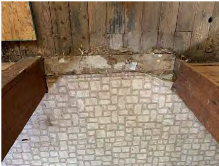
Non-historic sheet vinyl, over plywood (bottom of photo), over original wood flooring (top of photo).
