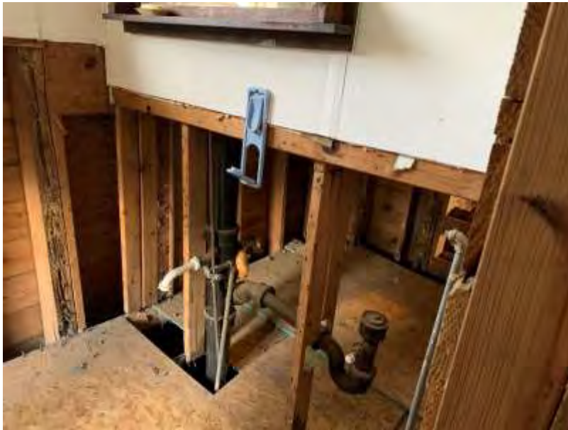
Cast iron waste plumbing in restroom area.
