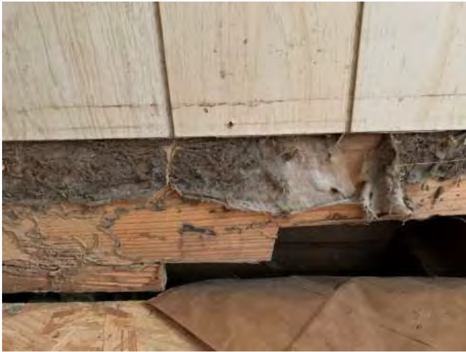
Remains of original wall papers backing under paneling.
