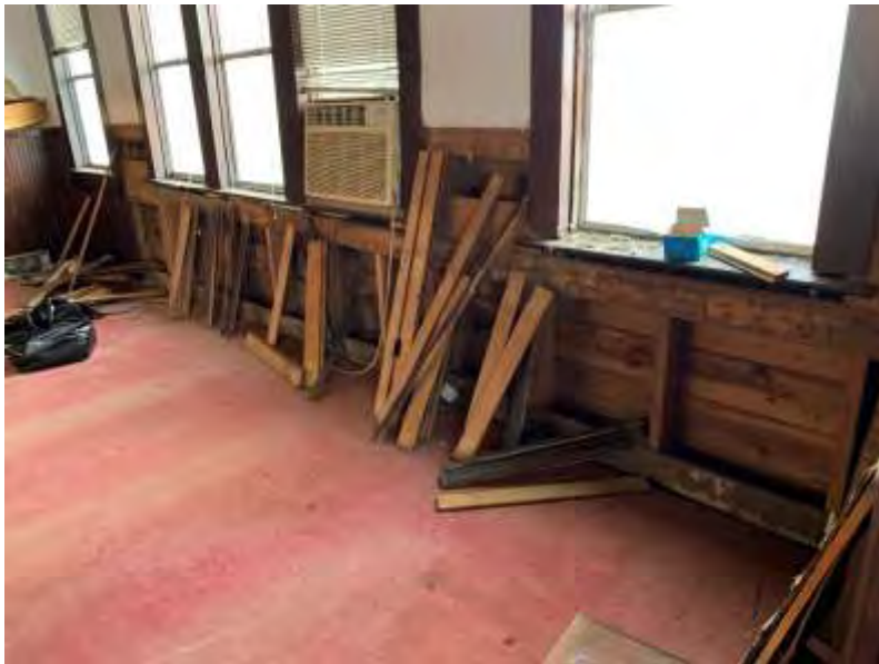
Sanctuary, west wall. Wainscot numbered and removed.
