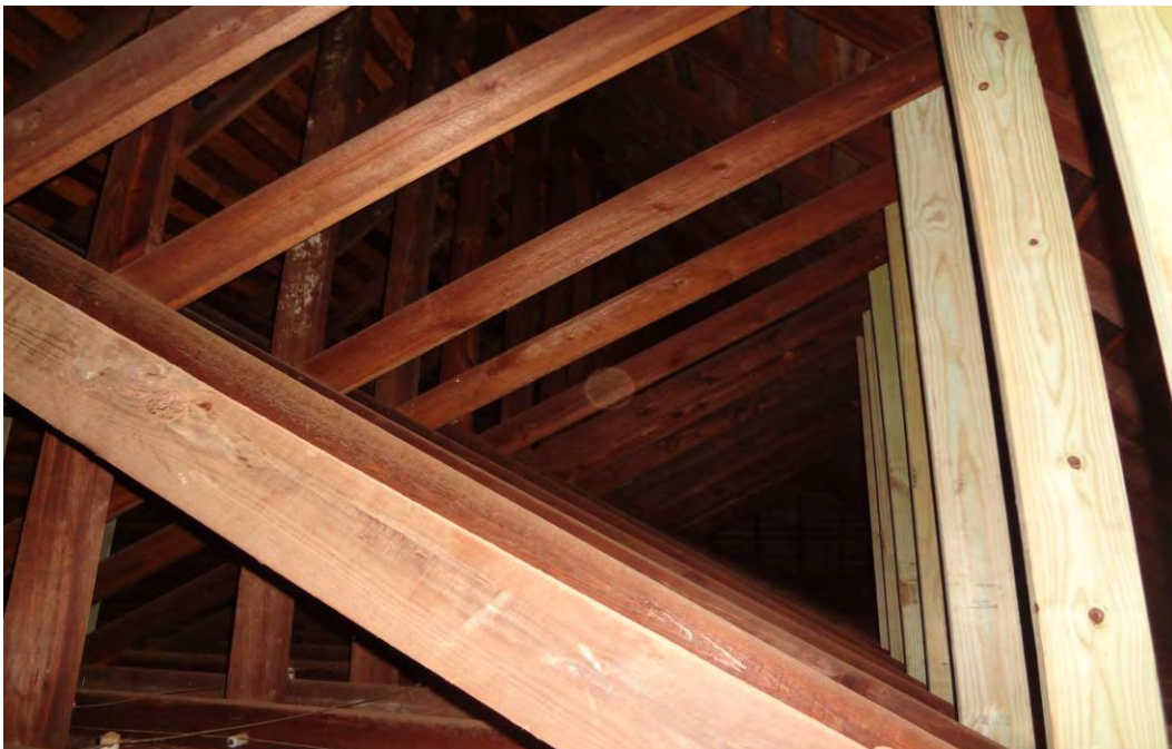
Photograph 4 – Typical Pony Wall Studs Attached to Top and Bottom Chords of Existing Roof Scissor Trusses.
