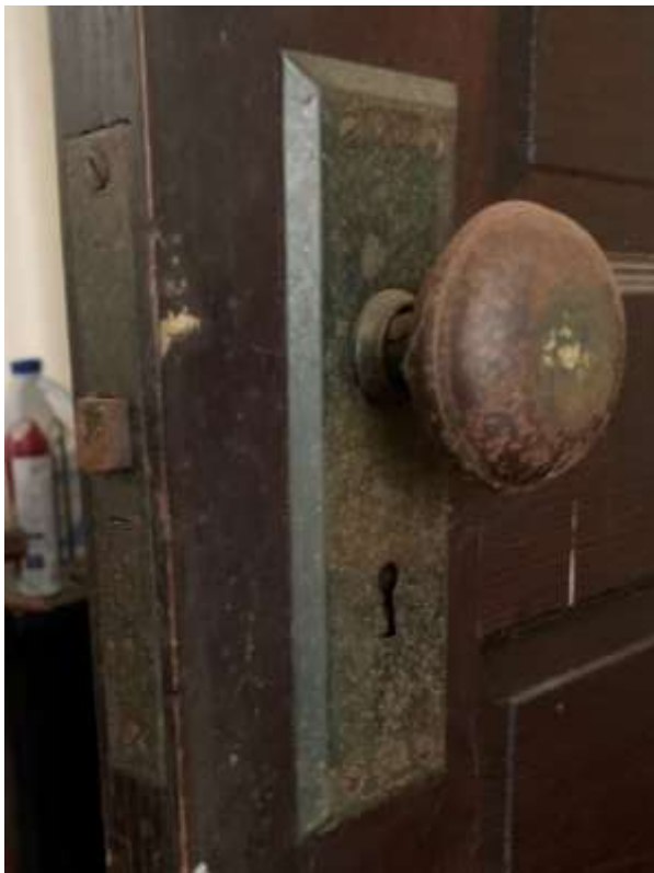
Typical original interior door latchset.
