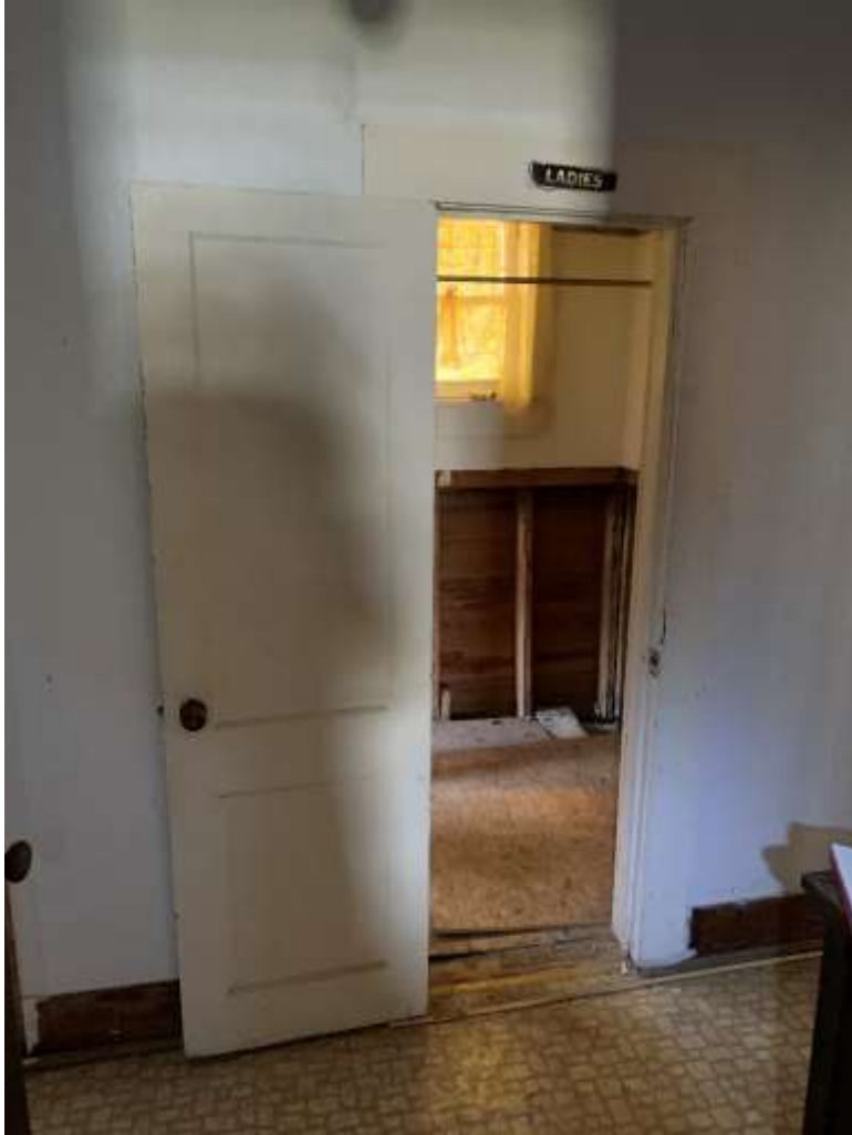
Narrow width, two panel door (24 inch Restroom door). Door and casings have been painted.
