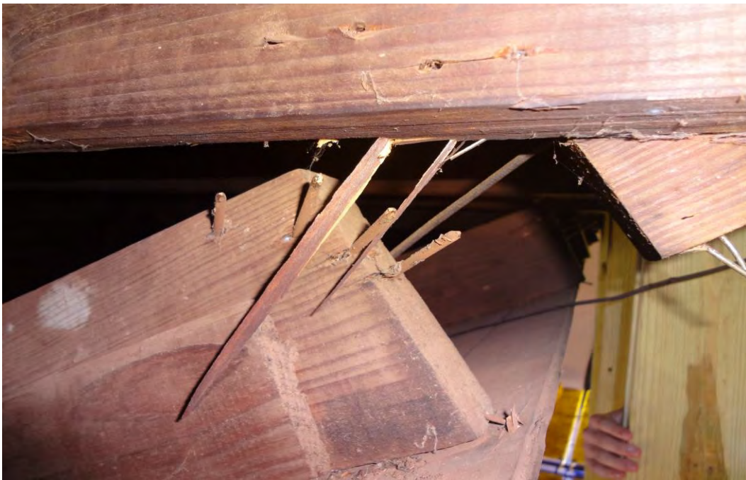
Photograph 6 – Typical Sloped Bottom Chord Connection Failure.
