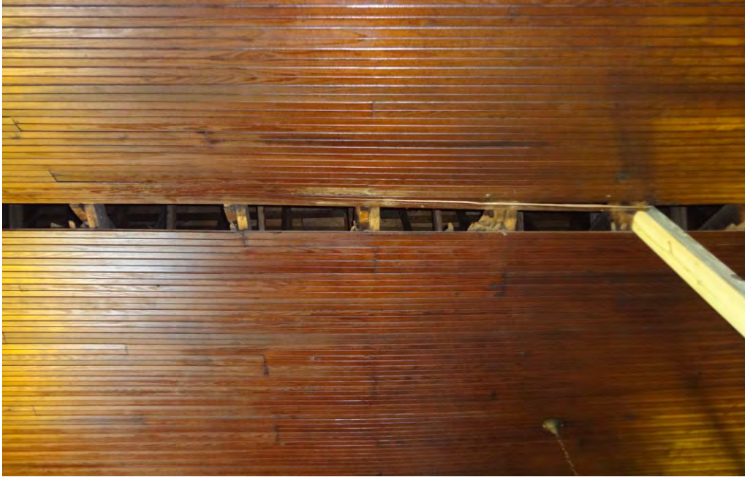
Photograph 3 – Typical Horizontal Bottom Chord to Sloped Bottom Chord Transition.
