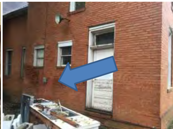
Former door location. Undetermined reasoning for previous configuration. Needs additional investigation. It is possible the original floor plans did not include indoor plumbing and the restrooms were added later.
