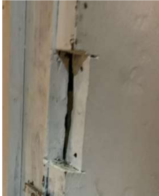
Ca. 1950's latchset. Evidence of removed rim latchset. Chiseled out casing for rim latch receiver.
