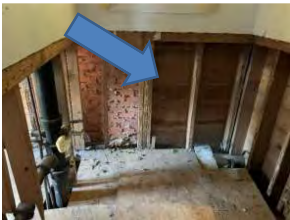
Former door location. Undetermined reasoning for previous configuration. Needs additional investigation. It is possible the original floor plans did not include indoor plumbing and the restrooms were added later.
