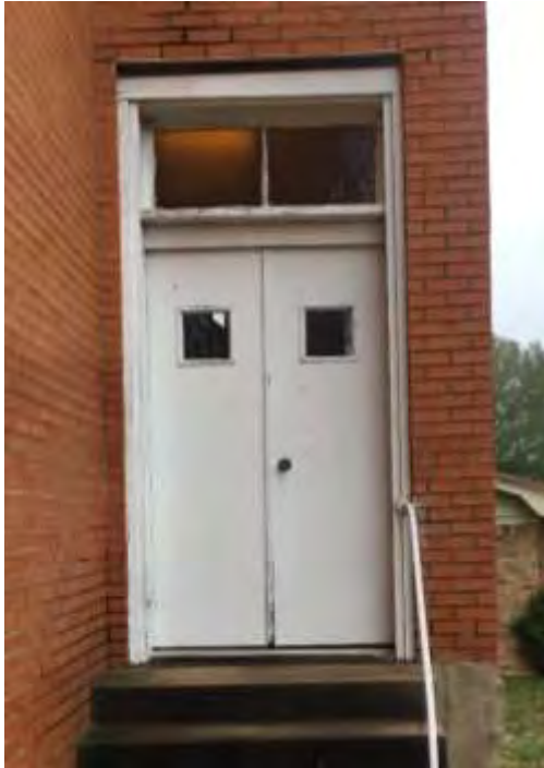
Southeast tower ca. 1950's door pair. Wood transom and frame are original.
