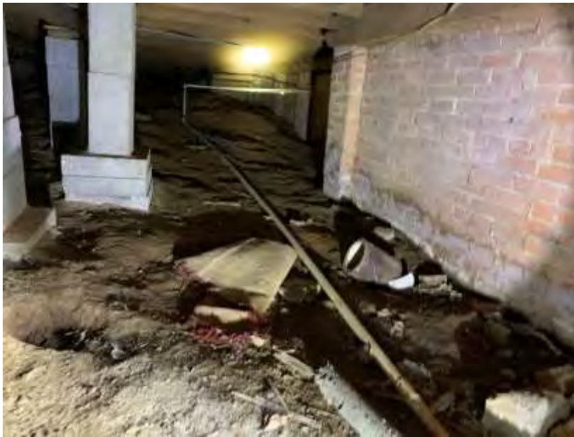
Crawl space. Presence of moisture along the east grade beam.
