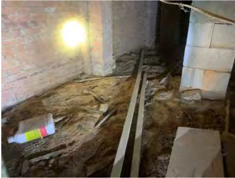
Crawl space. Evidence water had run along the south grade beam due to a previous heavy rain event.
