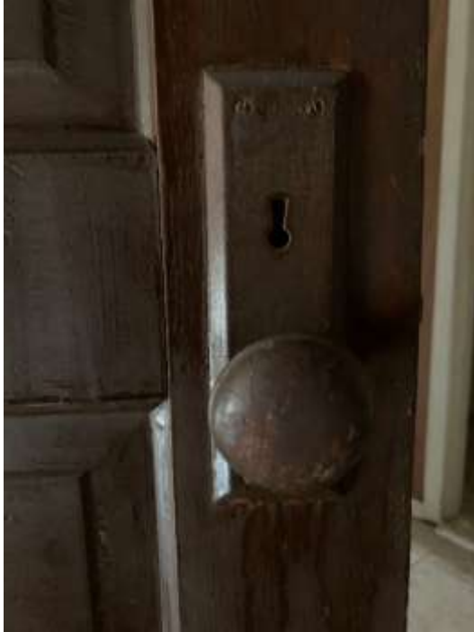
Original door hardware later reinstalled upside down.
