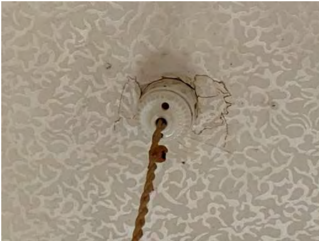
Ceiling paper and ceramic light fixture mounting base.
