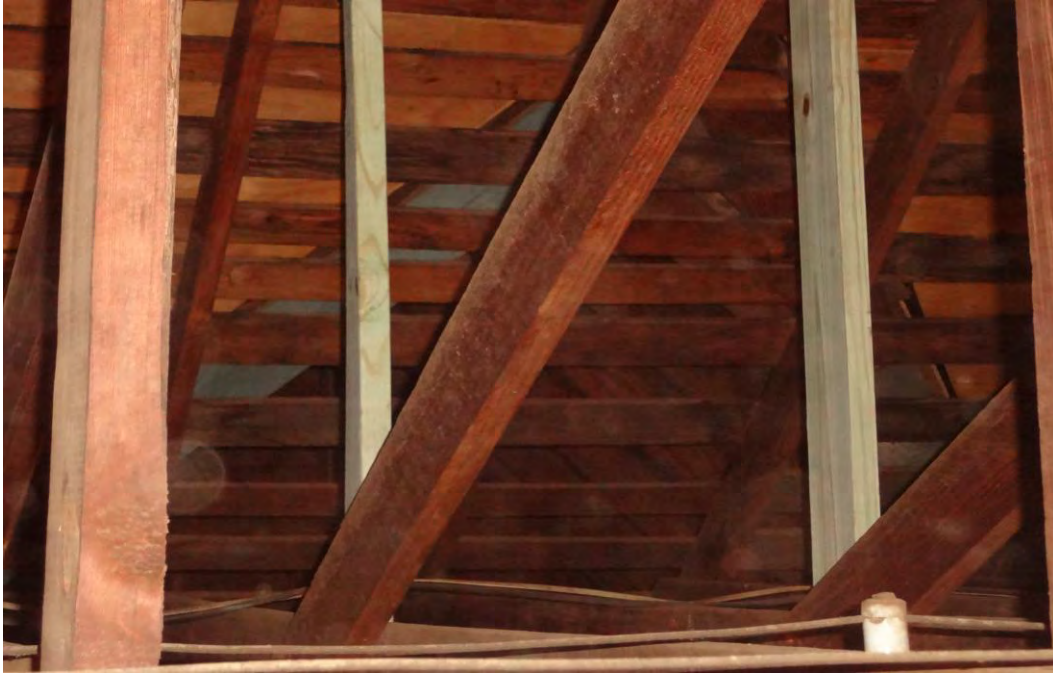
Photograph 5 – Typical Pony Wall Studs Attached to Top and Bottom Chords of Existing Roof Scissor Trusses.
