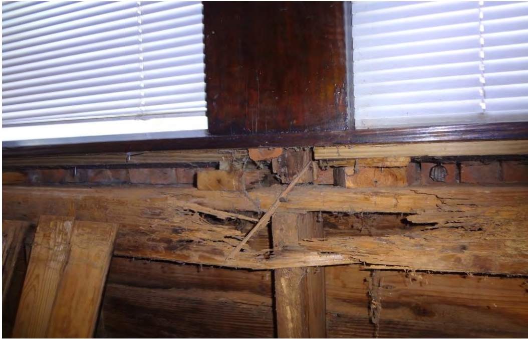
Photograph 1 – Typical Termite Damage at Windows along East and West Walls of the Sanctuary.
