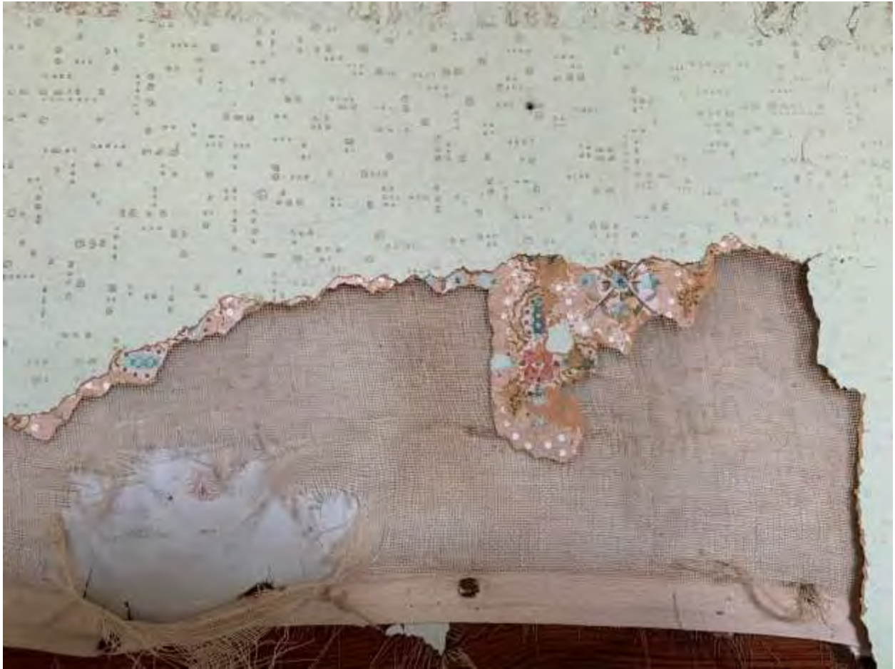
Two generations of wall paper. First layer of white is suspected of being an underlayment installed with the first generation cloth backing and floral paper.
