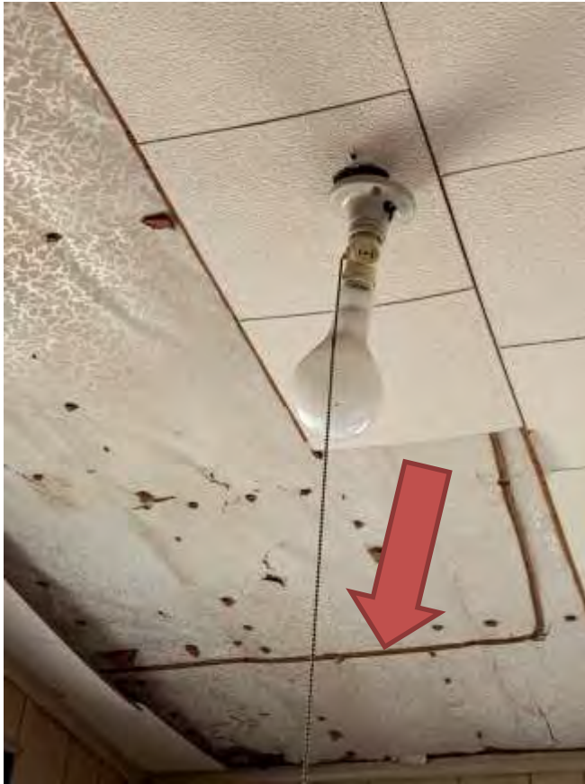
Wiring sandwiched between second generation ceiling wall paper and fiberboard ceiling tile.
