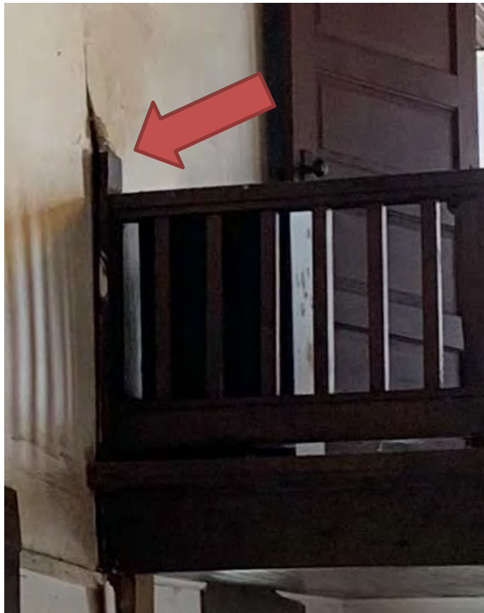
Balcony railing. Possible evidence of outward wall movement.
