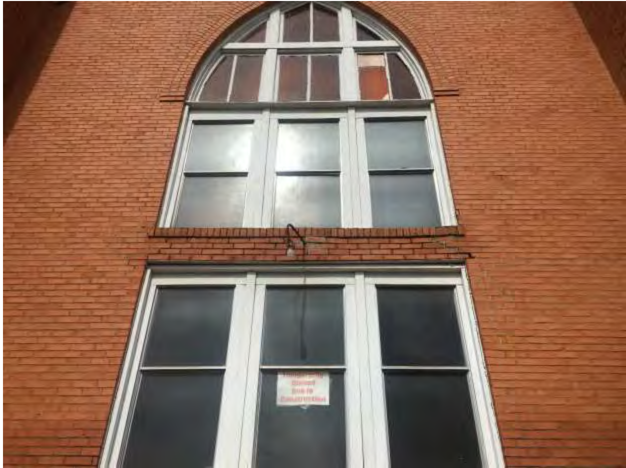
Upper gothic window is original wood framed. Six lower are aluminum. Typical for 3 locations of Sanctuary.
