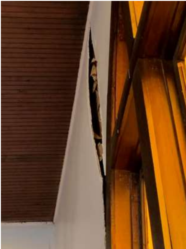
Sanctuary. Example of later added gypsum board damage due to outward wall movement and moisture.
