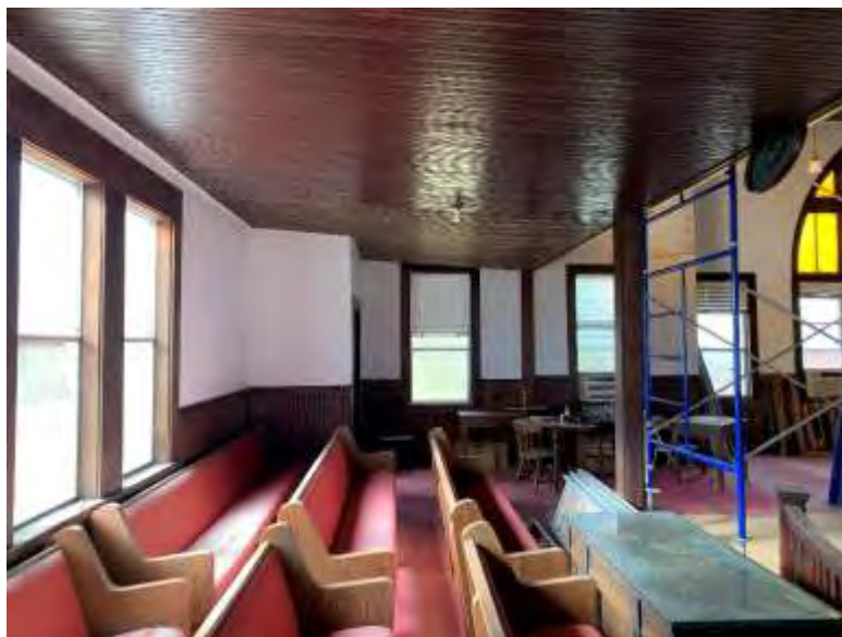
All lower, rectangular, windows of the Sanctuary are non-original aluminum frame.
