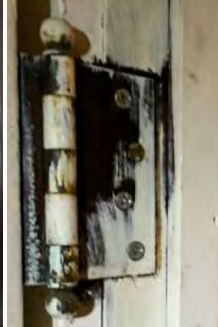
Original interior door hinge with remaining original finish. Modern replacement hinge.
