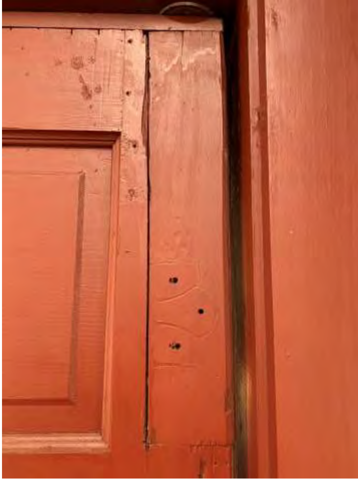
Crude repair to original door.
