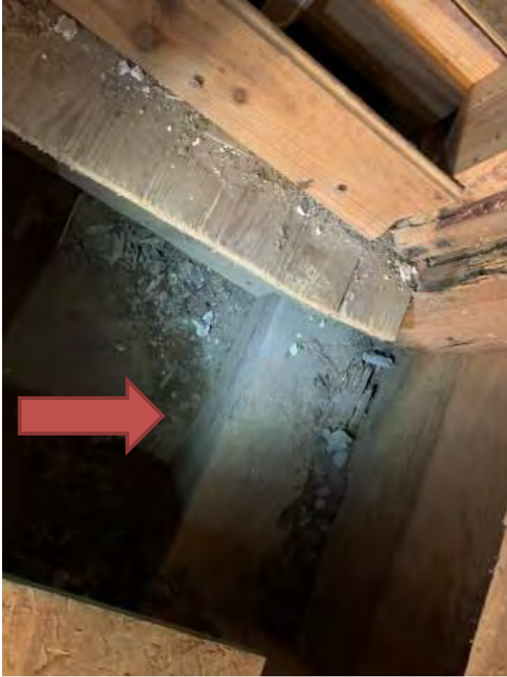
Near northeast corner at Women's restroom. Wood sill in contact with grade.
