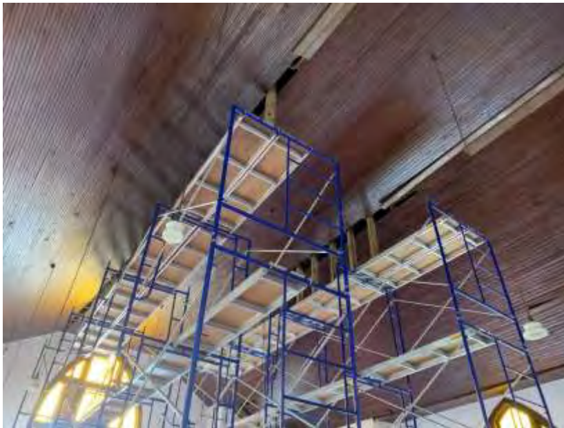
Sanctuary. Scaffolding erected to partially transfer roof loading.
