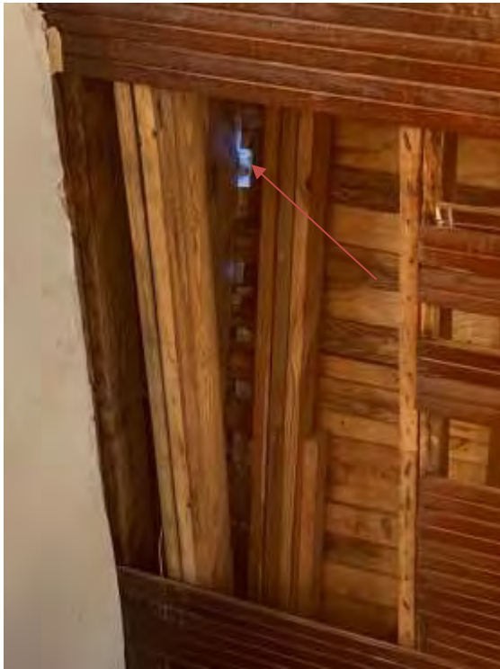
Example of roof opening where day light is visible from below.
