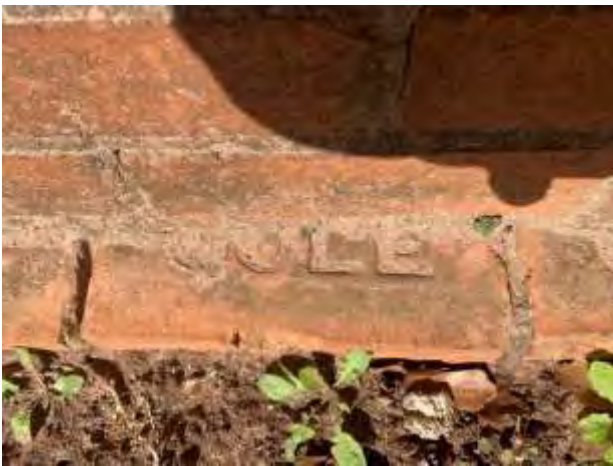
Exterior, west grade beam. The bottom of the grade beam appears to contain a corbeled brick footing in lieu of concrete as noted in the structural report.
