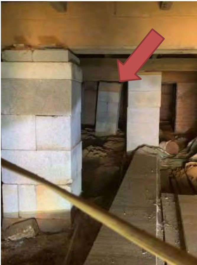
Crawl space, View to west. Several piers have settled and/ or rotated.
