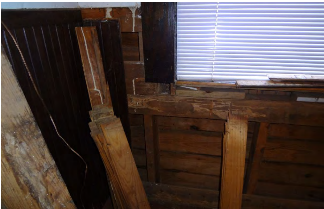
Photograph 2 – Typical Termite Damage at Windows along East and West Walls of Sanctuary.
