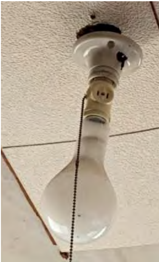
Ceramic base with bare bulb fixture.
