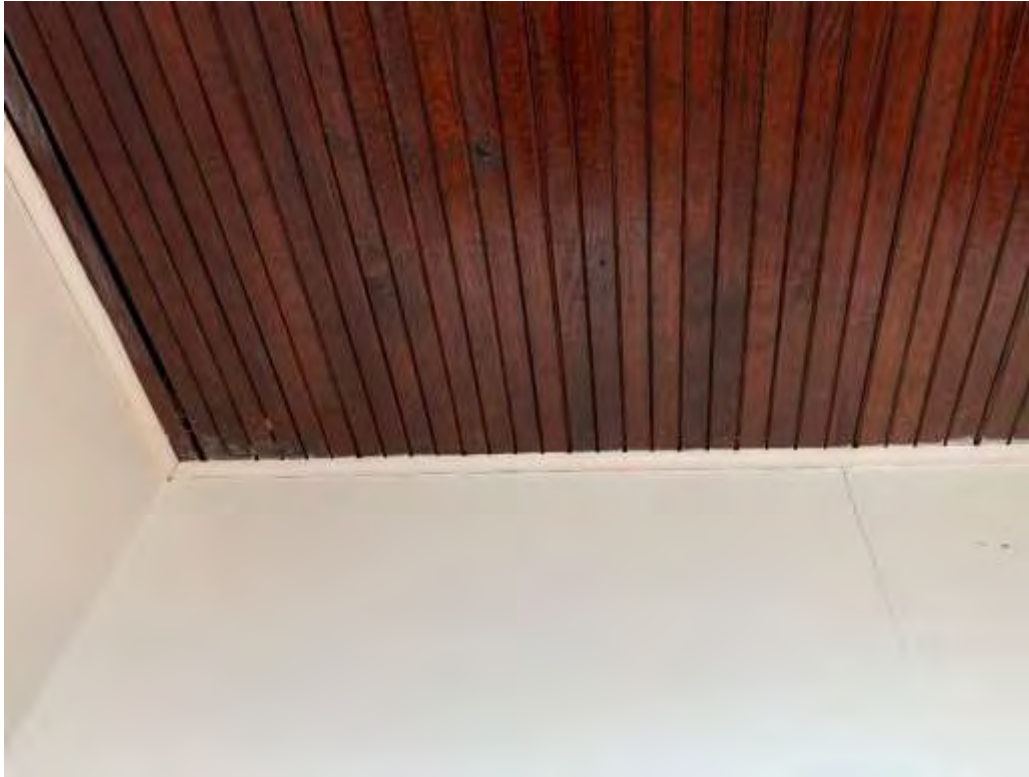
Beadboard ceiling with one generation of finish. Original moulding has been painted.
