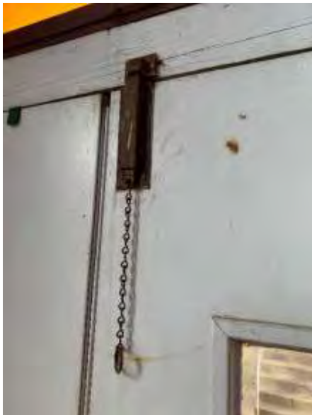
Probably a reinstalled original spring bolt (left) and modern knob on 1950's exterior door (right).
