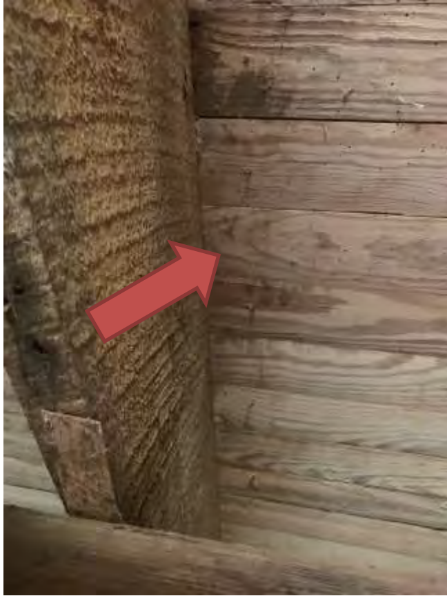
View upward from crawl space. Underside of long leaf pine flooring of Sanctuary.
