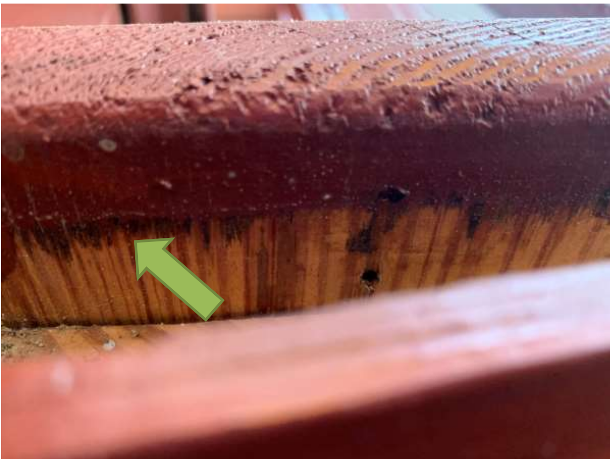
Residue of original wood finish.
