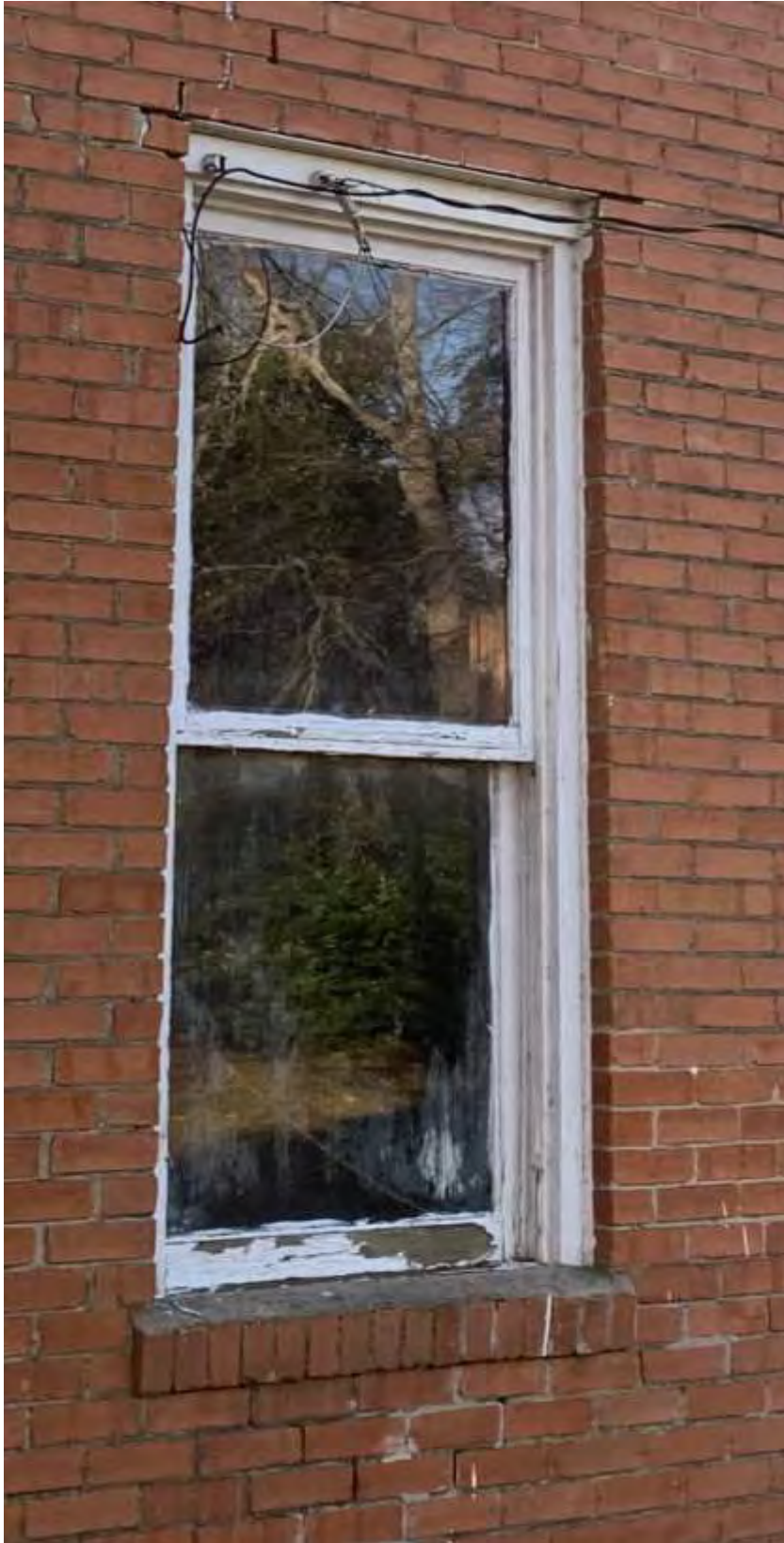
Example of original wood framed window with original glazing.
