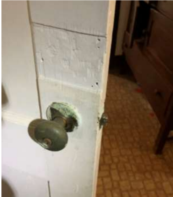
Ca. 1950's latchset. Evidence of removed rim latchset. Chiseled out casing for rim latch receiver.
