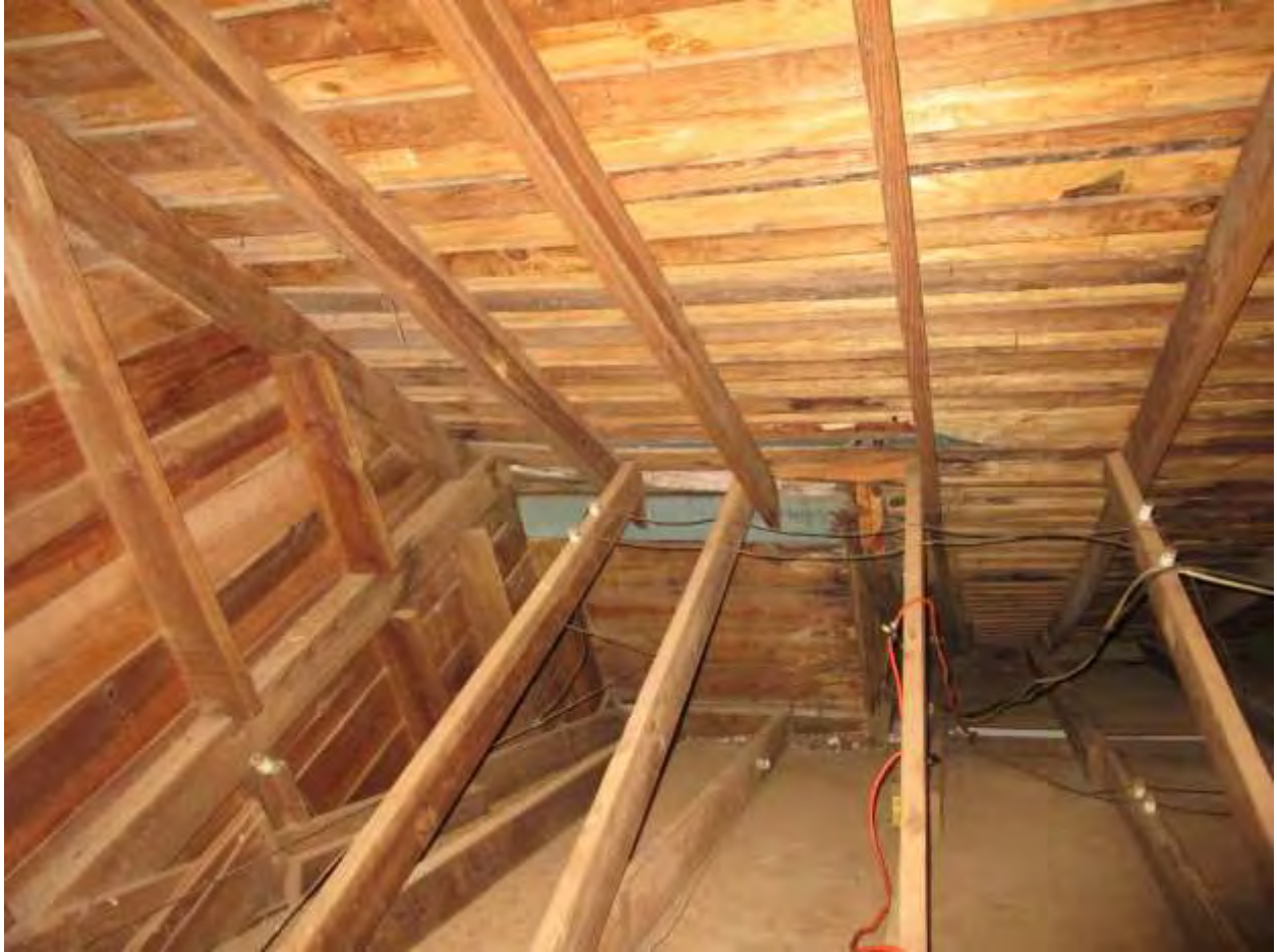
Attic, near southwest tower. Custom built scissor trusses.
