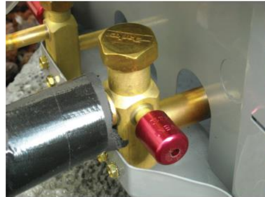
Refrigerant access port lock
