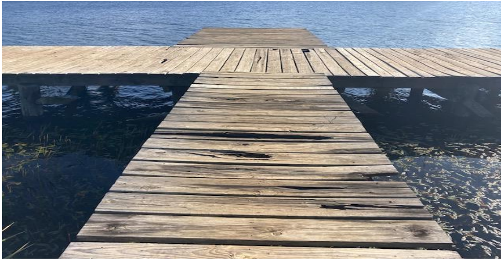
Damage to Fishing Pier Lower Lake
