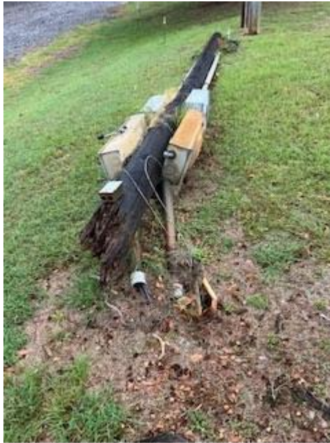
Broken Electrical Pole Spring Street and boxes
