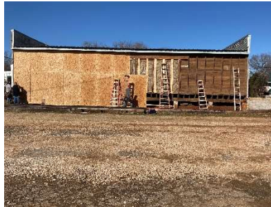
Installation of insulation and OSB
