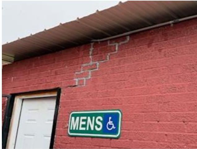
Bricks Reagan After Repair
