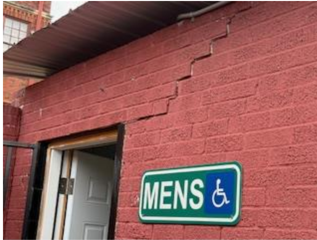
Brick Shift Upper Restroom Reagan Park Before
