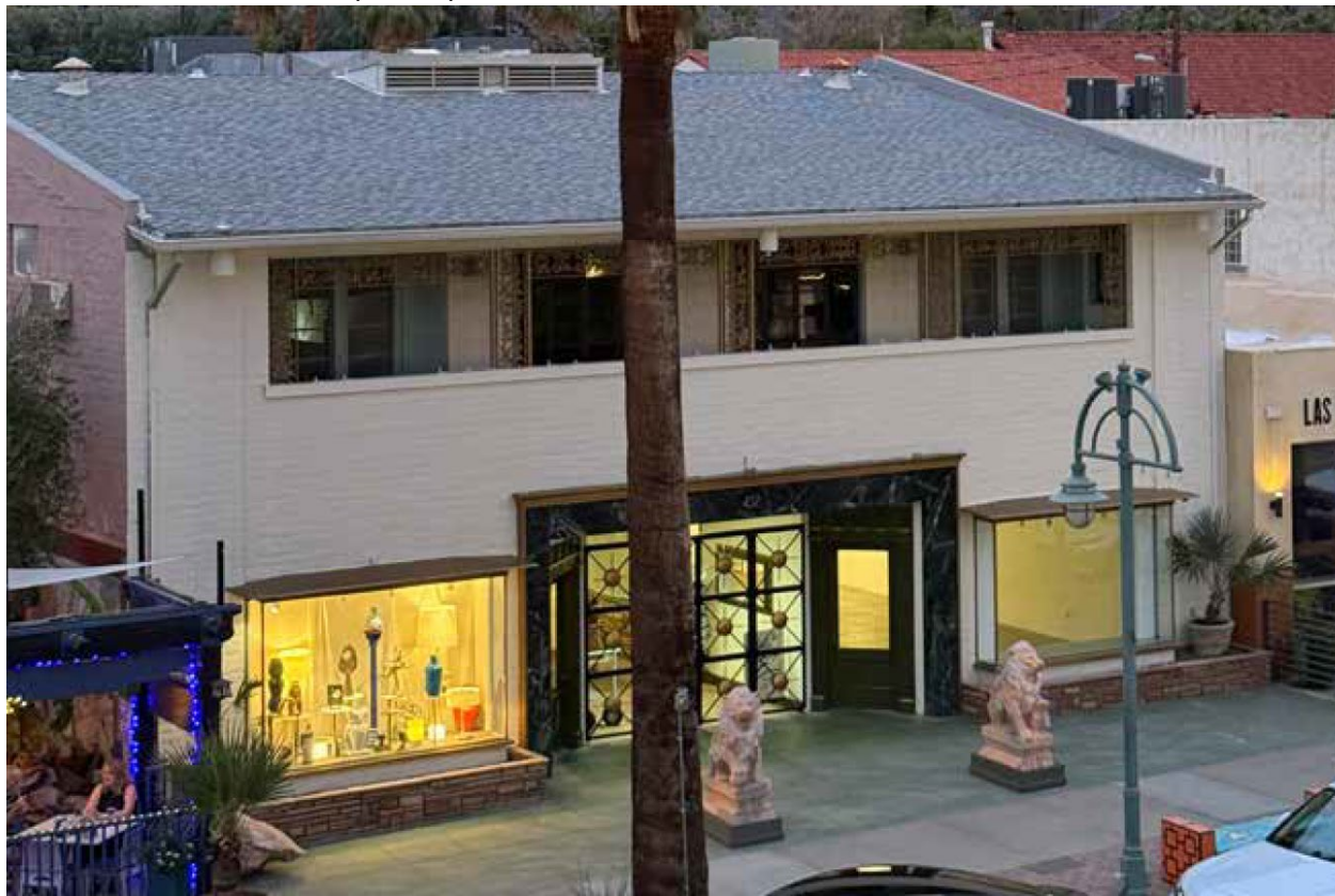
EAST (FRONT) ELEVATION FROM NORTH PALM CANYON, 2026.
