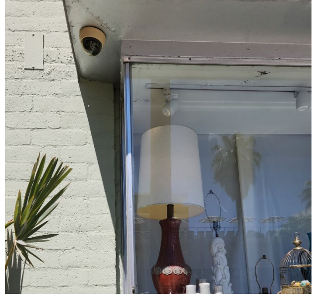
CLOSEUP PHOTO OF PAINTED SURFACE OF THE PROJECTING FRONT DISPLAY WINDOW
