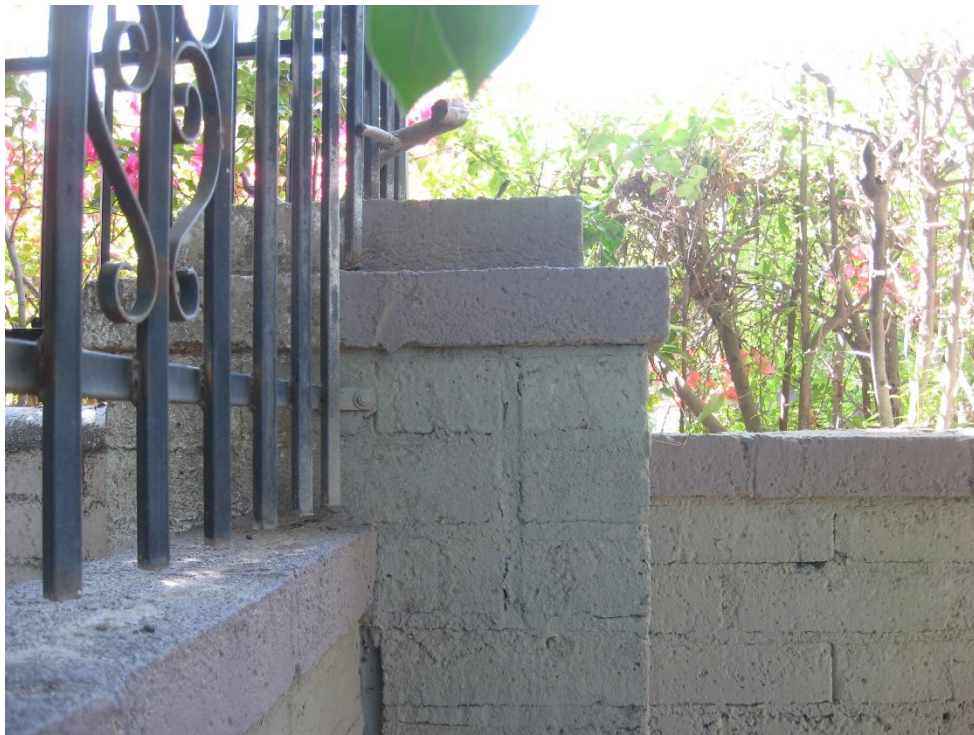
Detail of west perimeter wall showing original gate post of original 1932 driveway. (Author Photo. July 2023)
