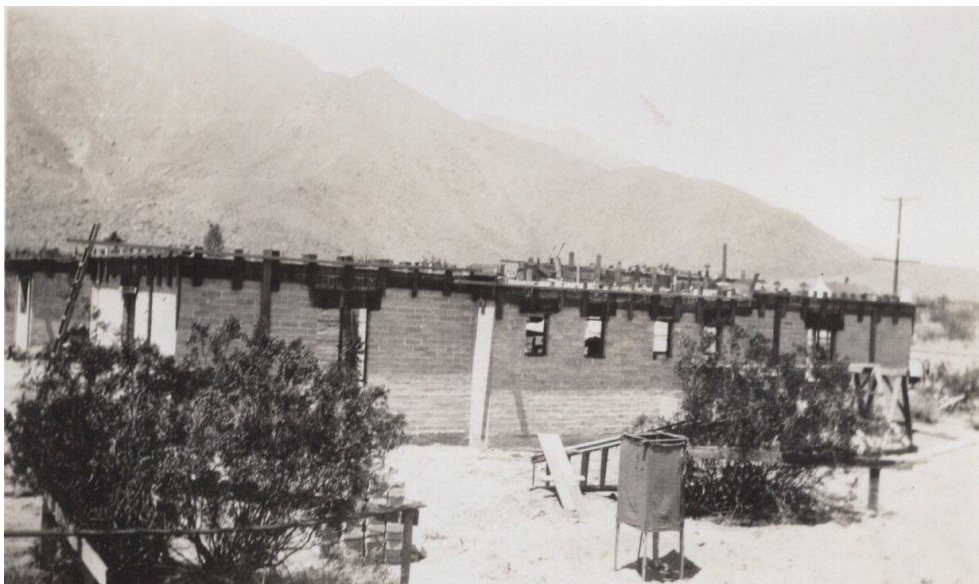
Construction photos ca. late 1931. Top view looking northeast. Bottom shows east façade. Note, quartet of windows.
