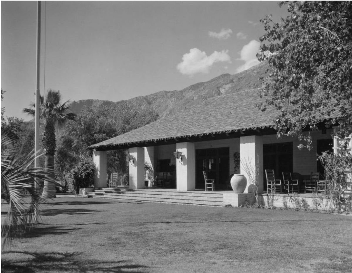
Nellie Coffman's Desert Inn, the hotel that put Palm Springs on the map was also William Charles Tanner's masterwork. There are numerous similarities between its design and that of Morada La Estrella. (Courtesy Mott-Merge Collection. California State Library)
