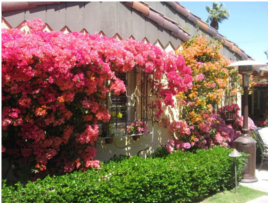
The steel window grilles, designed in traditional Spanish style, are not original features but are period appropriate. (Author photo. July 2023)
