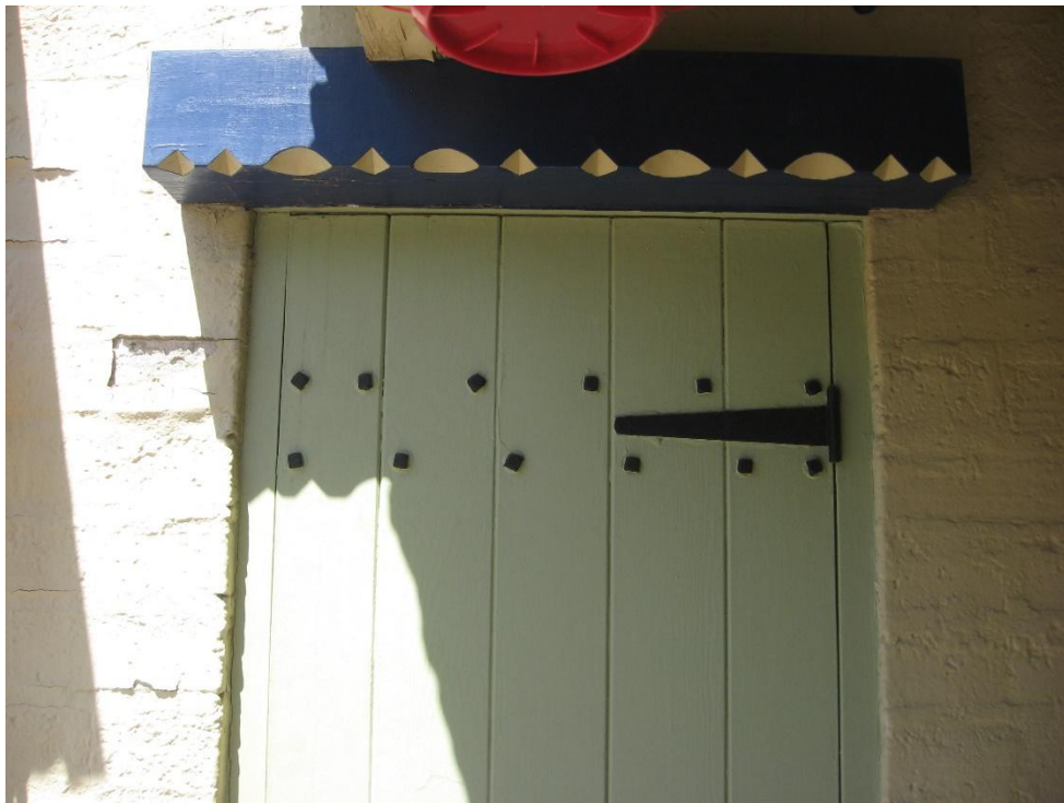
Detail of studded service door. Note carvings on lintel. (Author Photo. July 2023)
