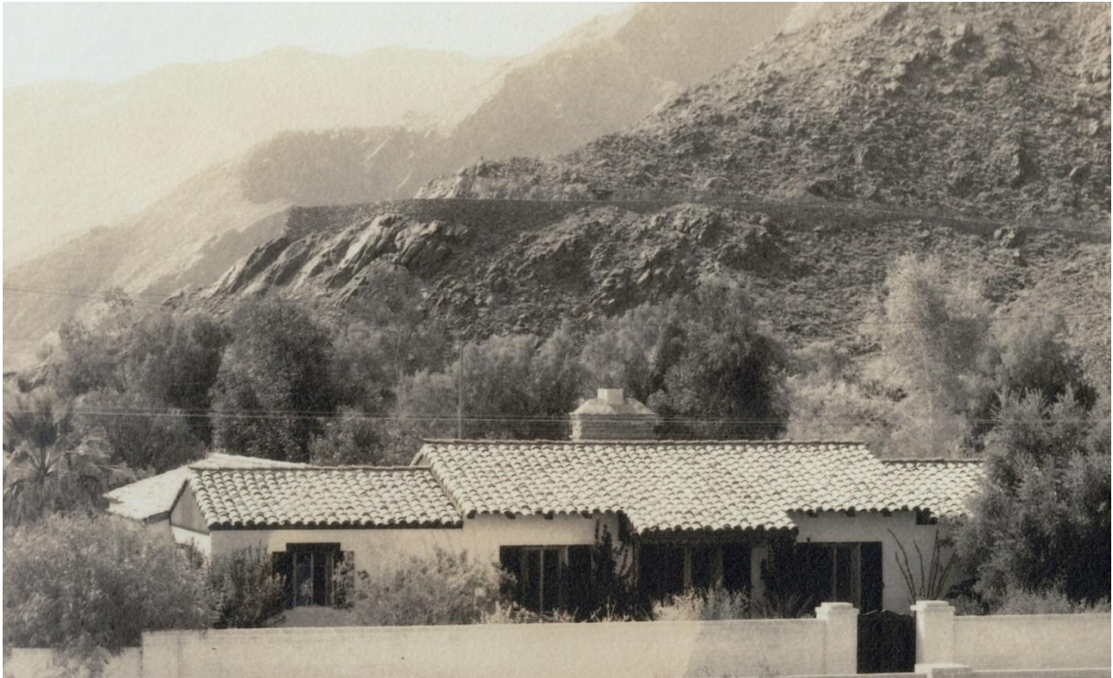
Tanner's use of varying roof pitches added visual interest to the low-slung massing of the house. Note, Inspiration Point on the mountain above. (Courtesy of Mary Kummings and Steve Scott)
