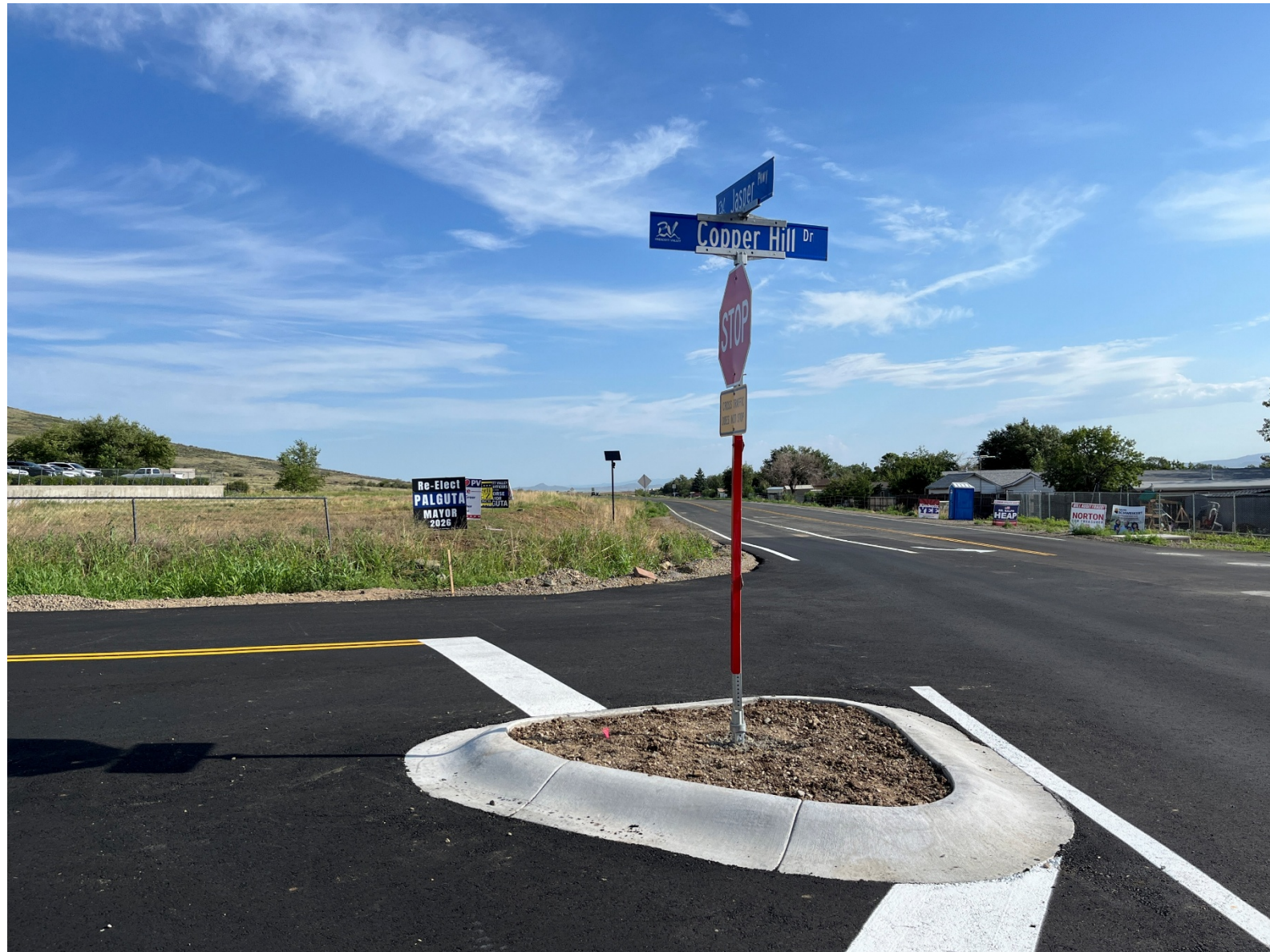
Jasper Parkway & Copper Hill Drive grade mitigation
