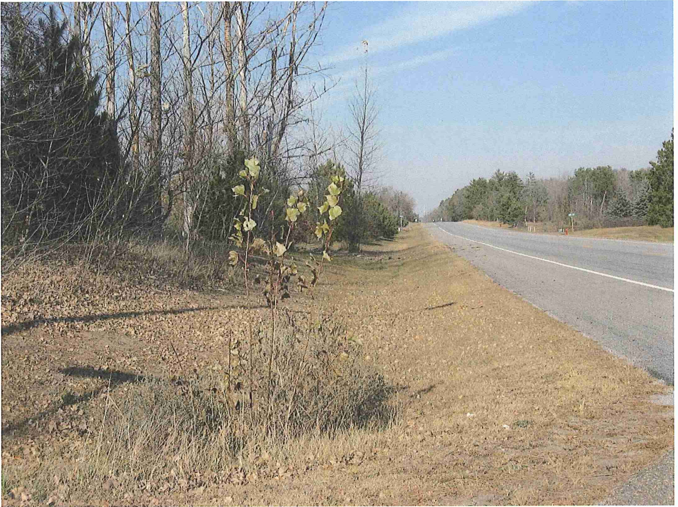
LOOKING NORTH ALONG VARIOLITE STREET FROM 157 TH AVE
