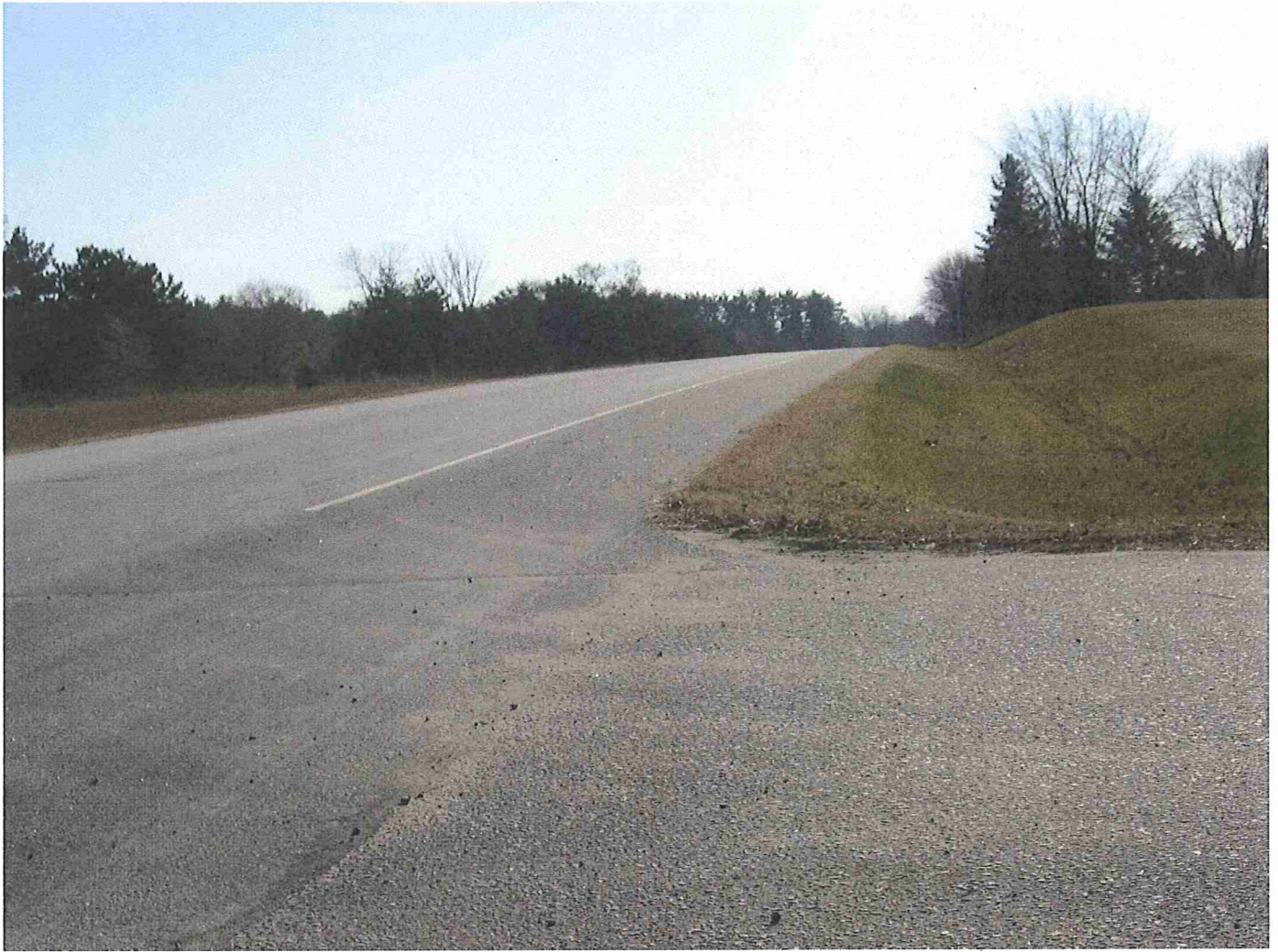
LOOKING SOUTH ALONG VARIOLITE STREET FROM 157 TH AVE.
