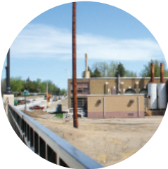
Hutchinson power plant
