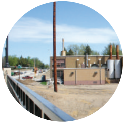
Hutchinson power plant
