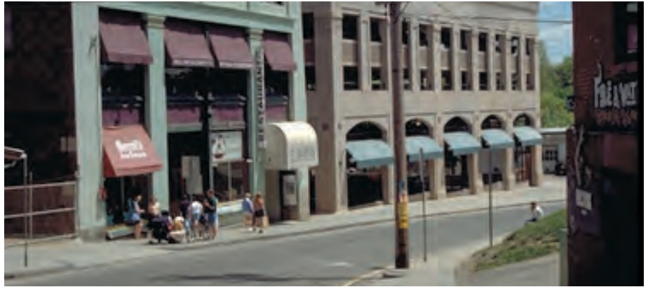
Parking ramp design (building on the right) includes awnings, arched openings and similar materials to reflect character of adjacent building.
