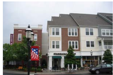
Window and door openings
