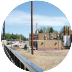
Hutchinson power plant
