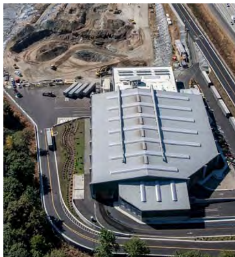
Bow Lake Transfer Station Aerial View
