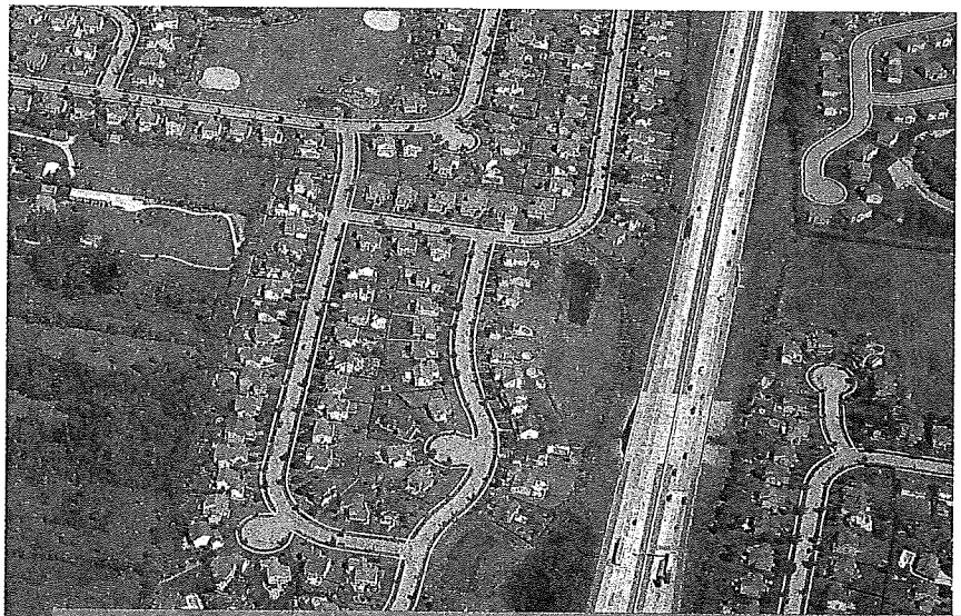
These images show how Pictometry images were combined using Photoshop to illustrate a new highway in Mundelein, Illinois.
