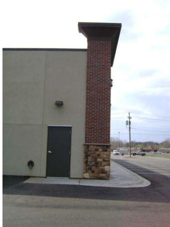
Sample Roof Screening
