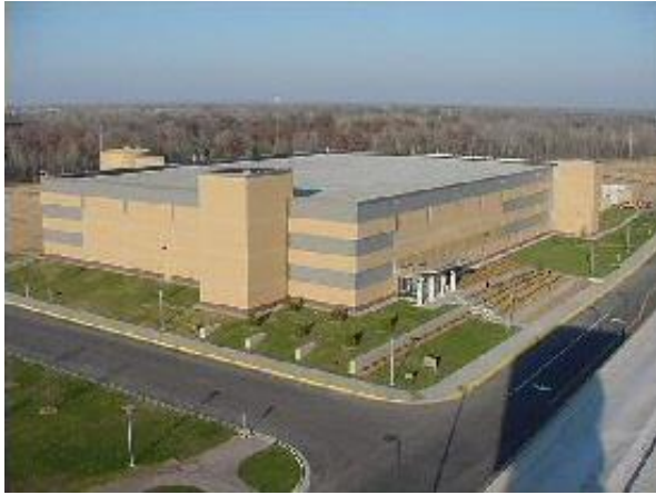
Target Data Center, Brooklyn Park
