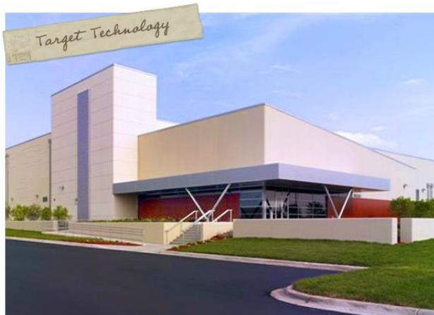
Target Data Center, Elk River
