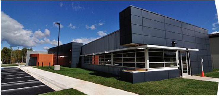
Involta Data Center, Duluth
