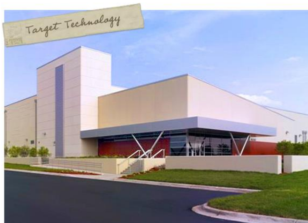
Target Data Center, Elk River
