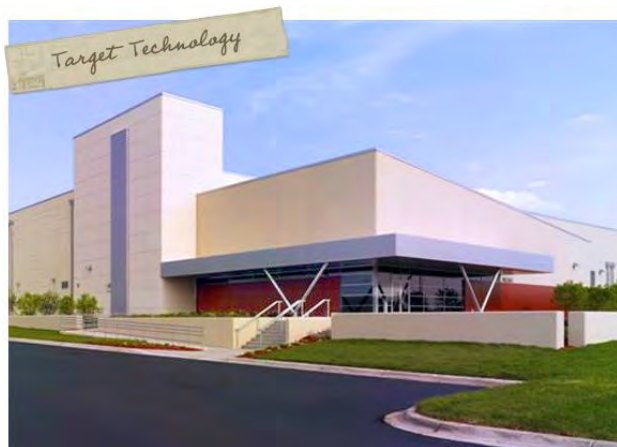
Target Data Center, Elk River
