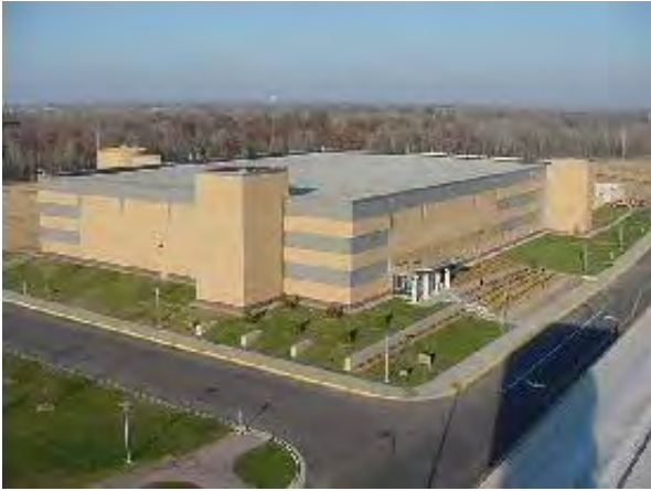
Target Data Center, Brooklyn Park
