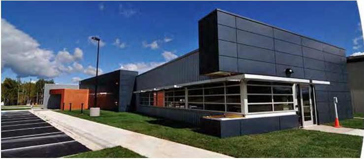
Involta Data Center, Duluth
