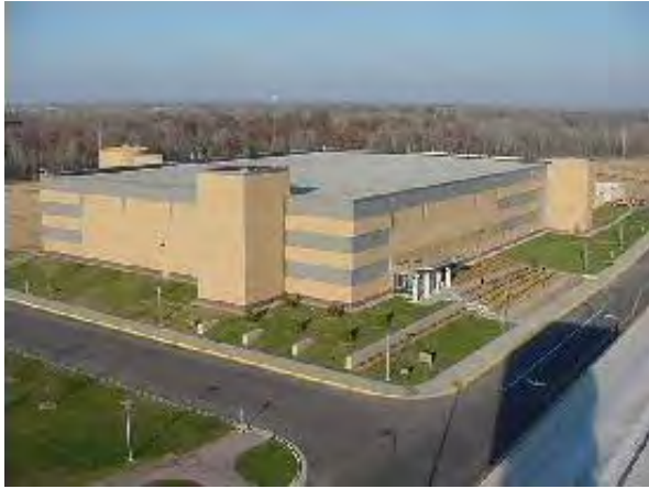
Target Data Center, Brooklyn Park
