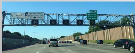
Overhead Lane Use Signs
