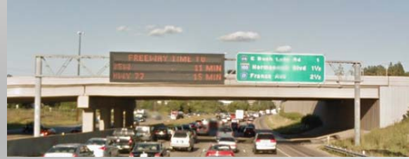
Overhead Dynamic Message Sign
