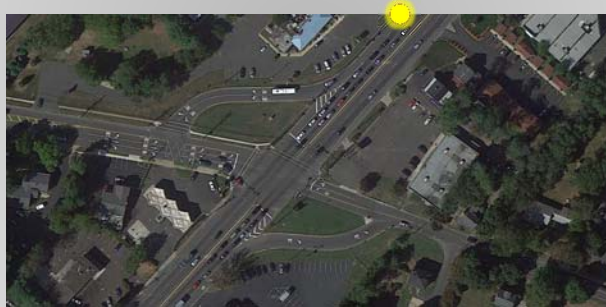
US-1 at Franklin Corner Road, Lawrenceville, NJ
