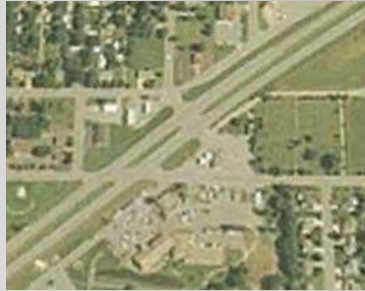
2004 Image of TH 169 in Belle Plaine, MN before driveway closure
