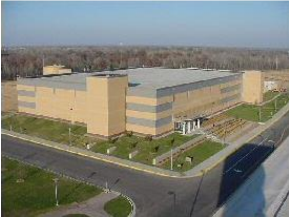
Target Data Center, Brooklyn Park
