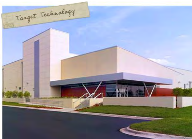
Target Data Center, Elk River
