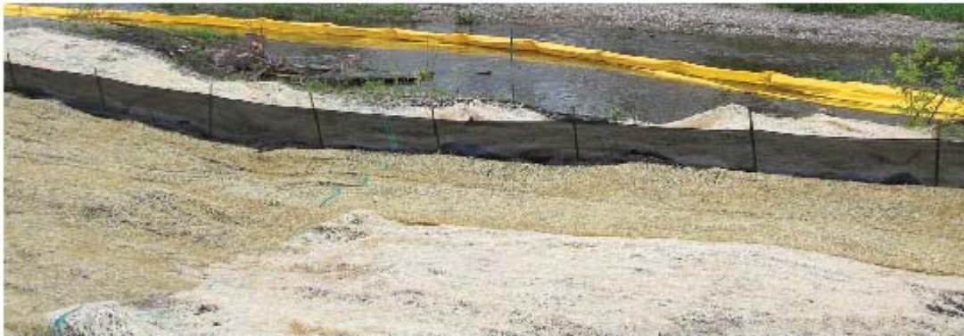
Areas near wetlands, lakes, watercourses or rock outcrops are likely habitat for reptiles and amphibians and may not be suitable for plastic mesh erosion control materials.
