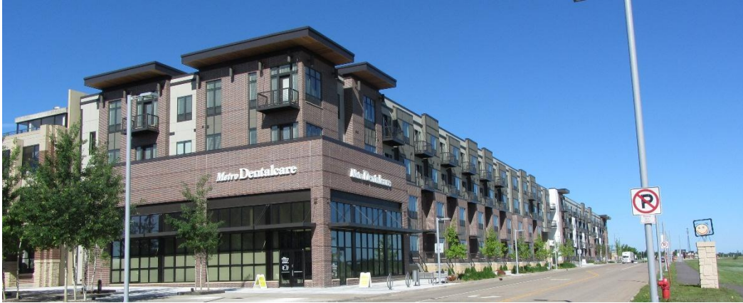
The above photo of Residence at the COR was taken August, 2013 along Sunwood Drive looking west.
