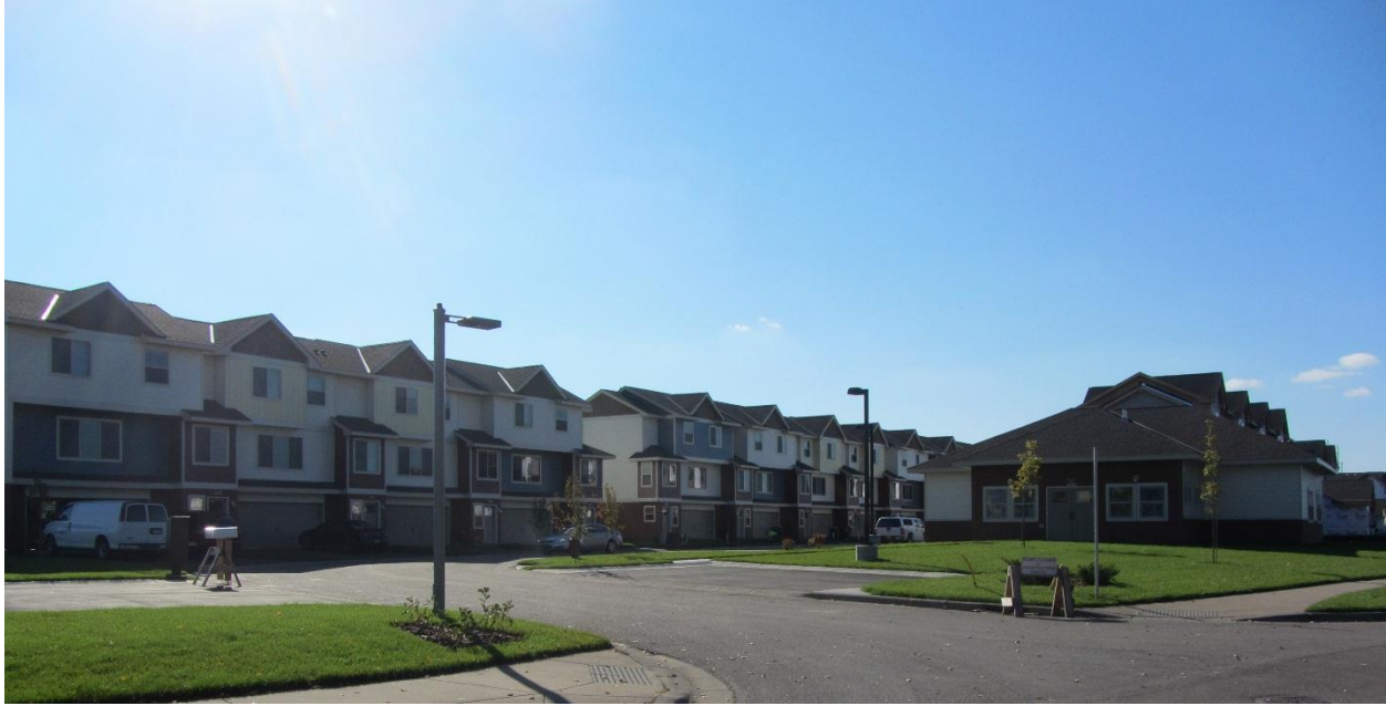
Photo taken on October 16, 2013 from 147 th Lane looking southwest.
