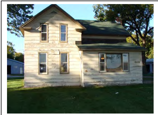
Existing home adjacent to CR 63 to be remodeled
