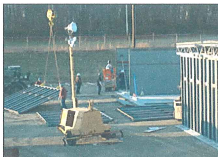
Alpha Range™ being installed on-site
