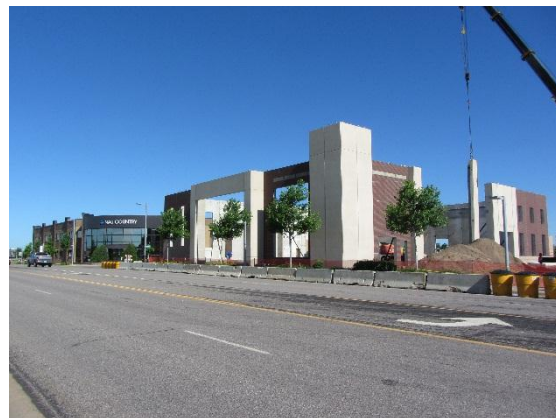
Photo taken June 20, 2013 at Sunwood Drive and Peridot Street looking north west.
