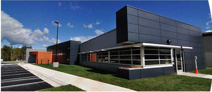
Involta Data Center, Duluth
