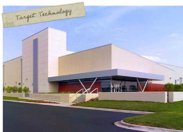
Target Data Center, Elk River
