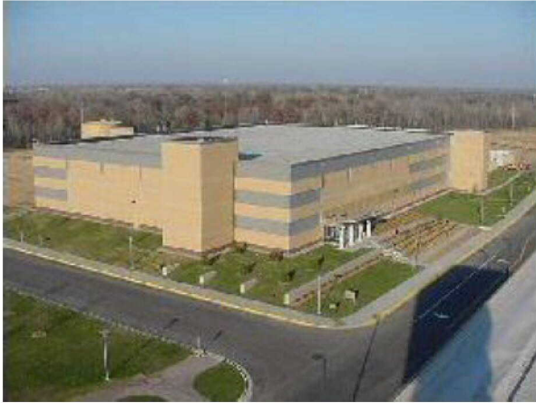
Target Data Center, Brooklyn Park
