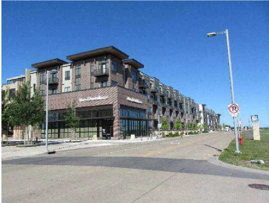
Photo taken June 27, 2013 along Sunwood Drive at the Municipal Center looking west.
