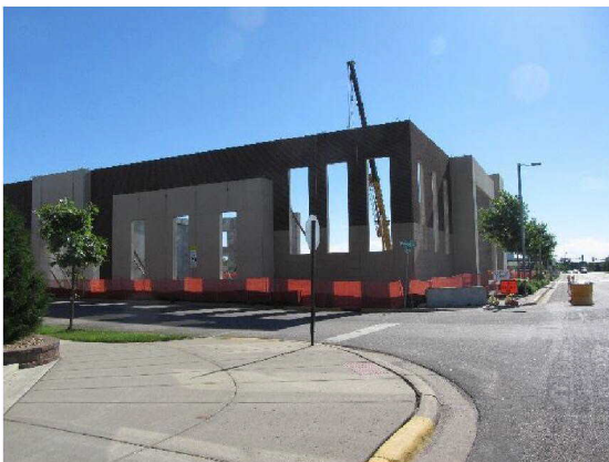
Photo taken June 27, 2013 at Sunwood Drive and Peridot Street looking north east.
