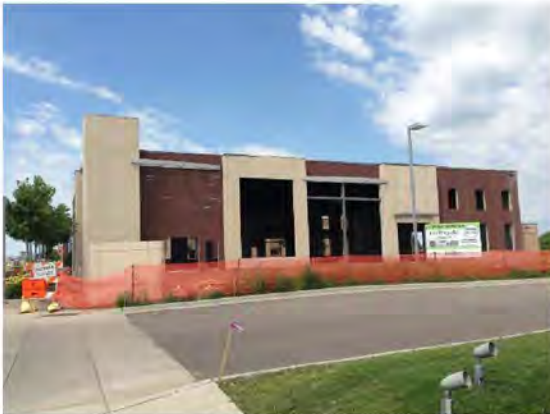
Photo taken August 1, 2013 at Sunwood Drive and Peridot Street looking north west.
