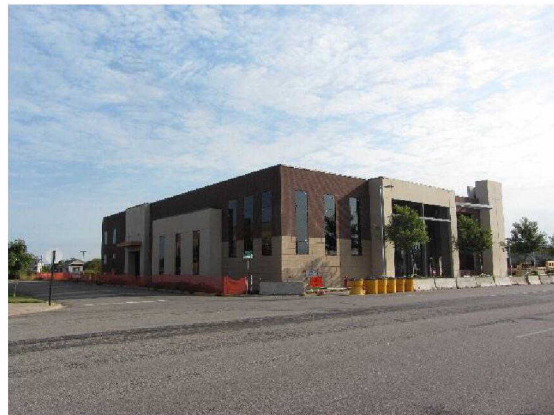
Photo taken September 5, 2013 at Sunwood Drive and Peridot Street looking north east.
