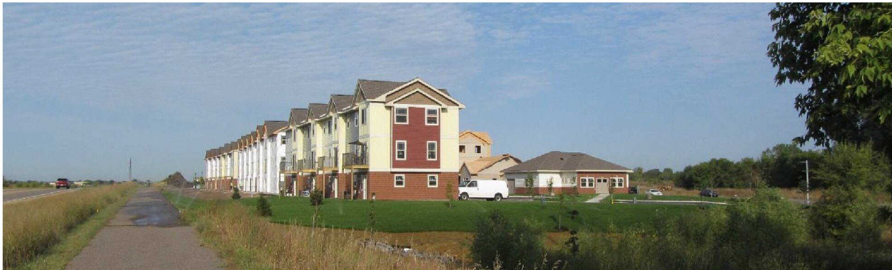
Photo taken on September 4, 2013 on the north side of Bunker Lake Boulevard looking west.
