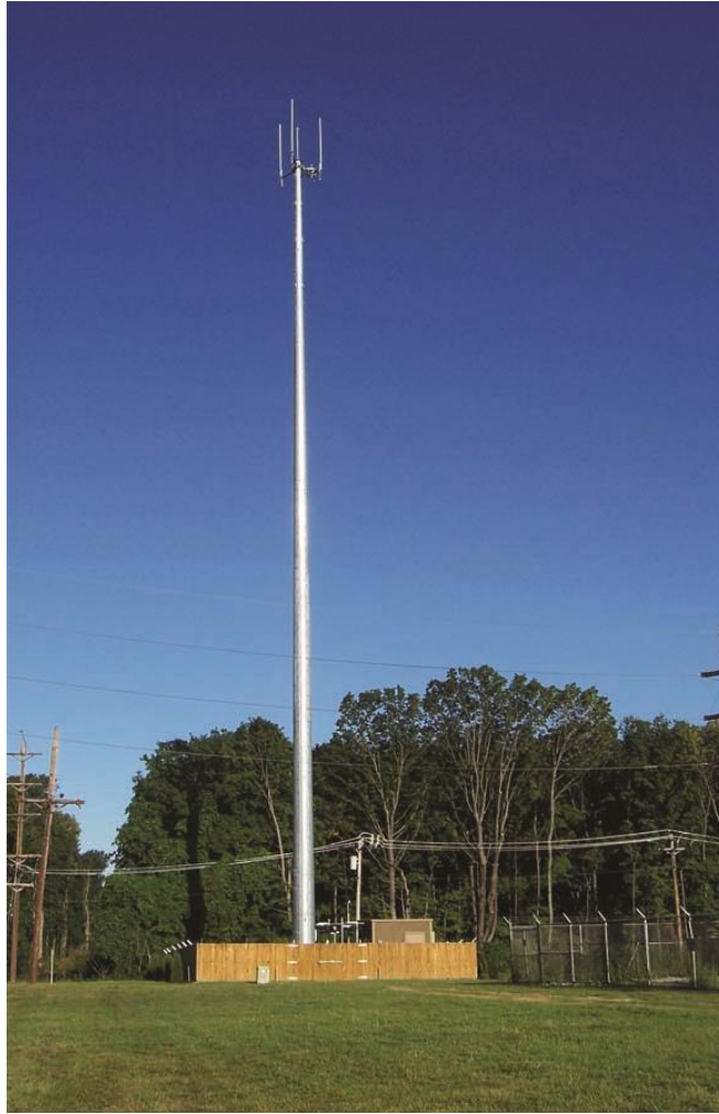
Exhibit 1: Similar monopole structure
