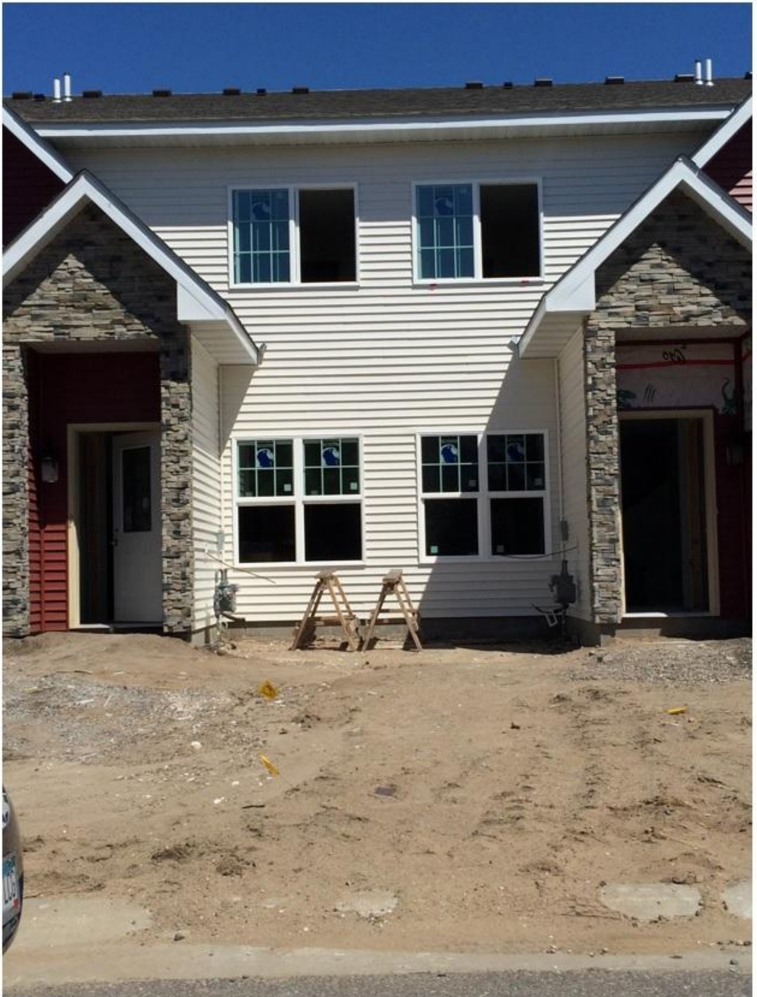
Ramsey Town Center Gardens 3 rd Addition Lot 3 Construction Site
