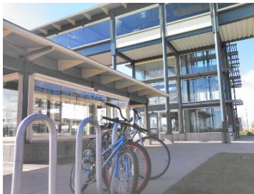
Ramsey Station, October 2014: People use the rail and bus service for commuting, efficient access to the airport, as well a connection to the region's trail systems
