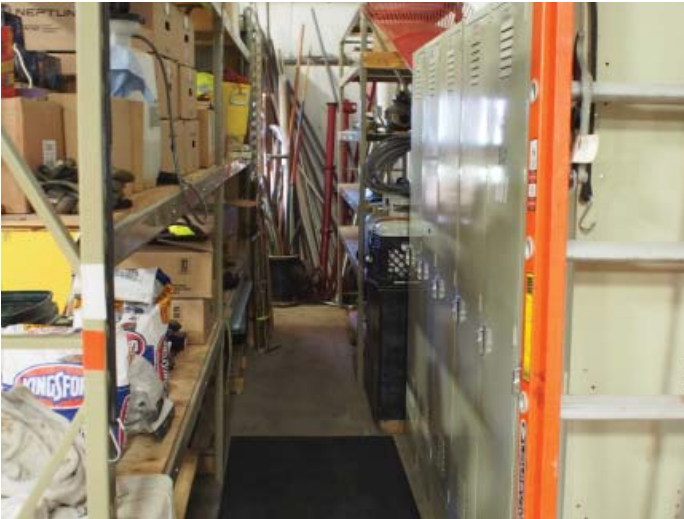
Figure B.I.11: Storage shelving placed too close together for safe access
