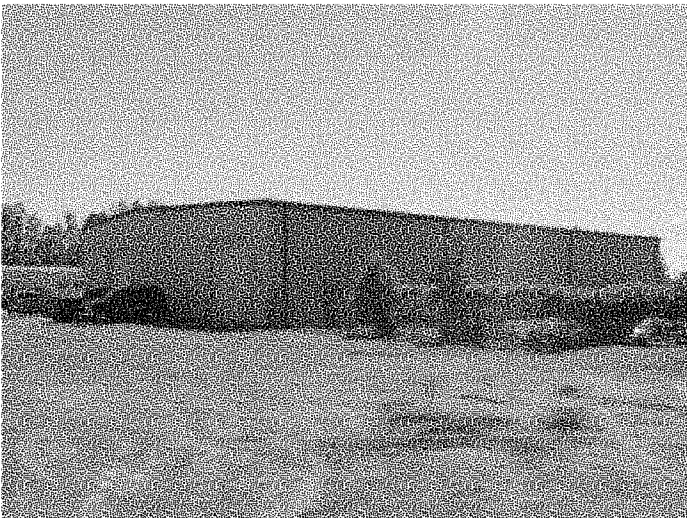
Figure B.2.1: Overall view of Cold Storage Building
