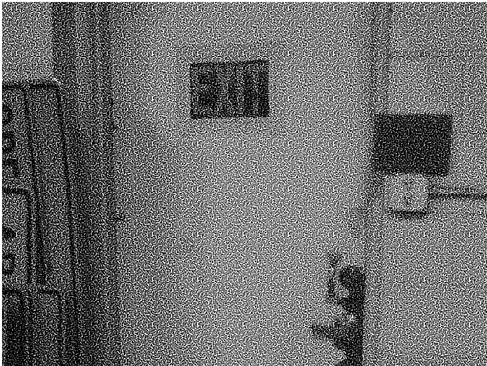
Figure B.1.12: Exit door has deadbolt with thumb-turn which is not allowed by code
