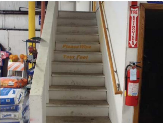
Figure B.1.13: Sign shop is not handicap accessible
