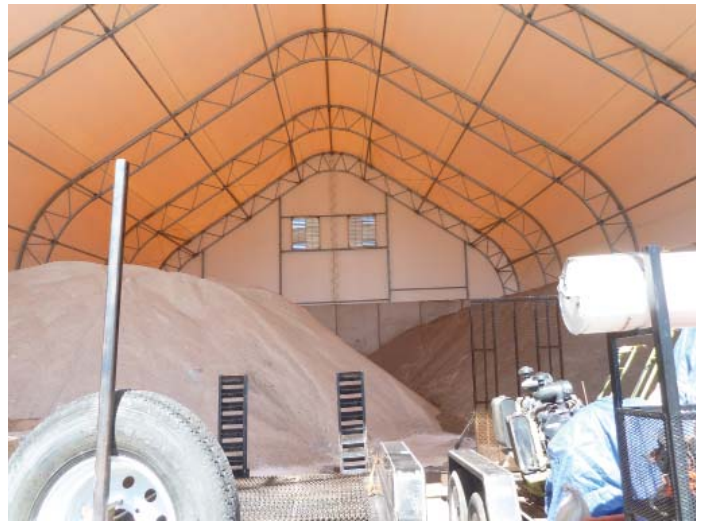
Figure B.4.3: Aluminum space frame structure appears in good condition
