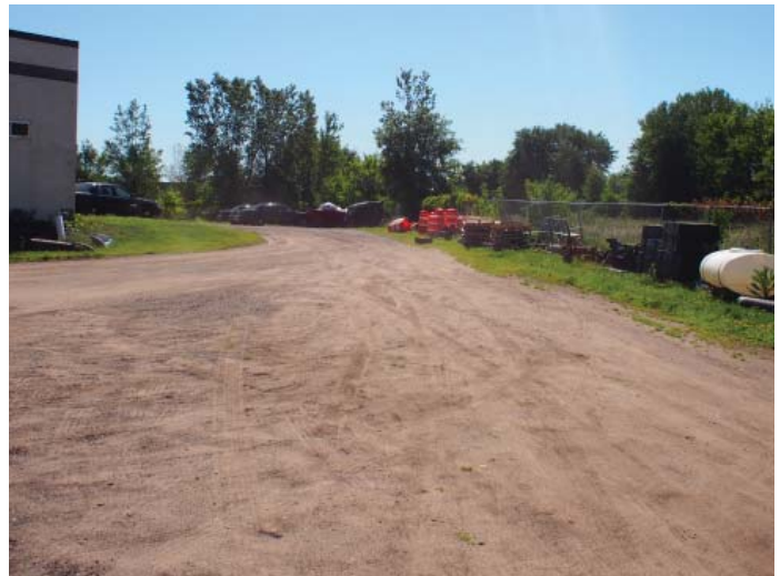
Figure B.6.4: Unpaved areas of site are in good condition with no signs of deep rutting
