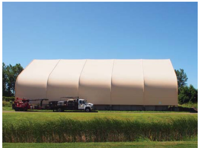
Figure B.4.4: Overall fabric roof structure is in good condition
