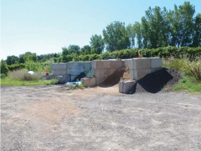
Figure B.6.6: Granular material storage bins are in good condition
