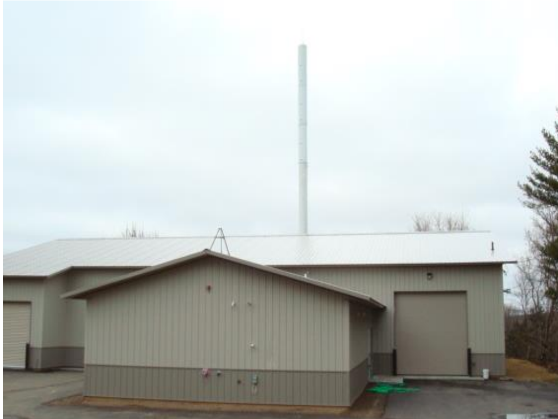
75' Canister Pole – Stillwater, MN
