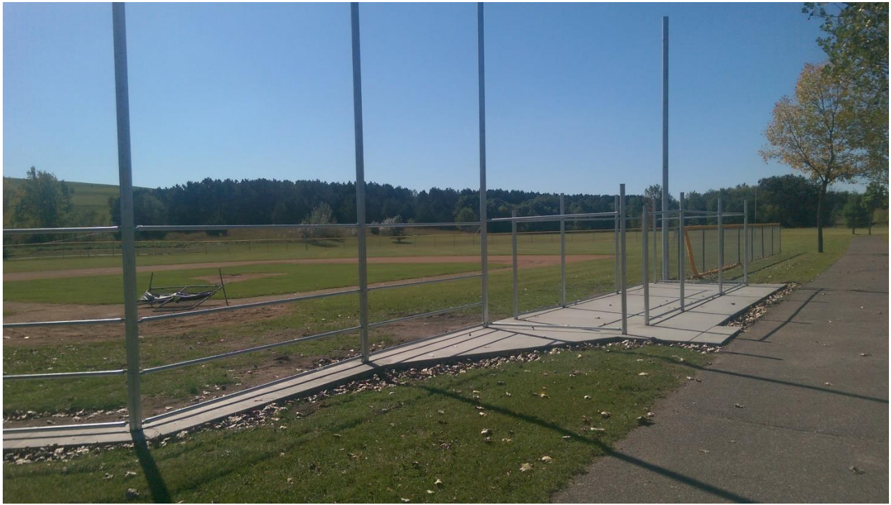
Ballfield #4 under re-construction — September 2017
