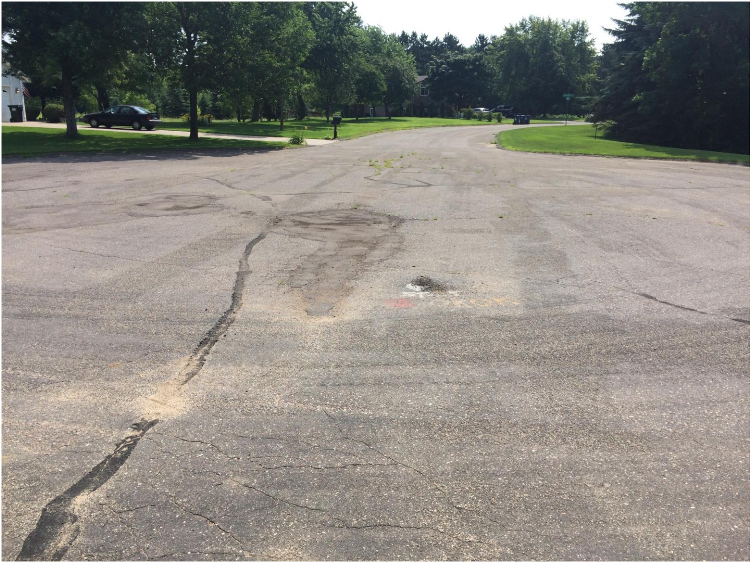
2: 164 th Lane cul-de-sac from West
