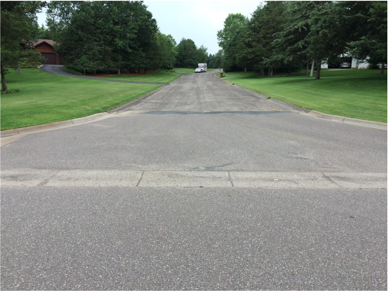
3: 154th Lane from Roanoke Street
