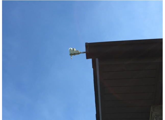
PROPER INSTALLATION OF A RAIN SENSOR
