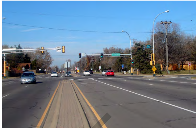
Roadway in Anoka County (Source: Anoka County)
