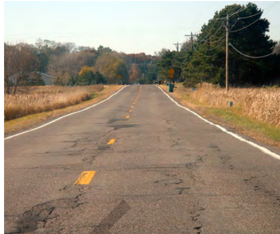
Roadway in Anoka County (Source: Anoka County)
