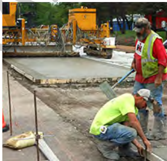
Reconstruction of an Anoka County Roadway (Source: Anoka County)
