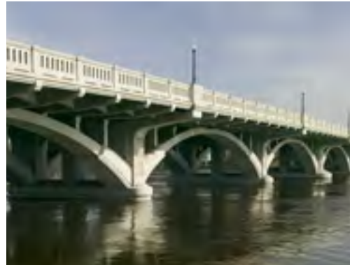
Anoka-Champlin Mississippi River Bridge (Source: MnDOT)
