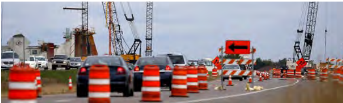
Construction Zone on Highway 10 in Ramsey (Source: Carlos Gonzalez)
