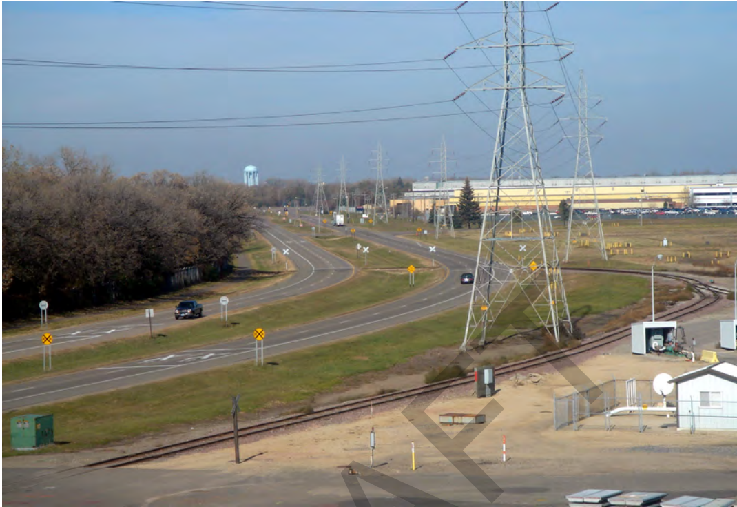
Freight Facility in Anoka County (Source: Anoka County)
