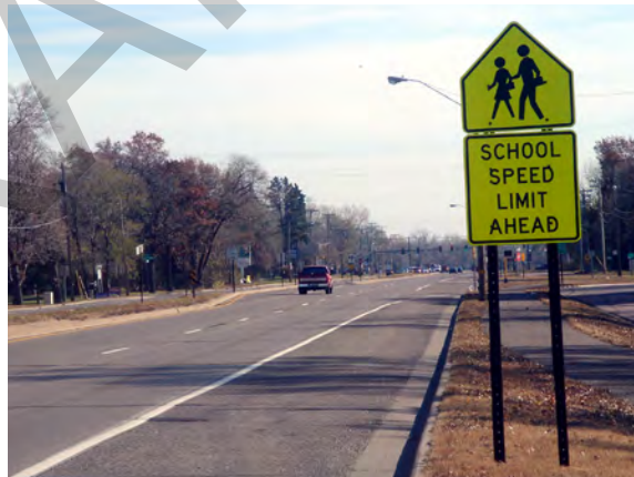
Roadway in Anoka County (Source: Anoka County)
